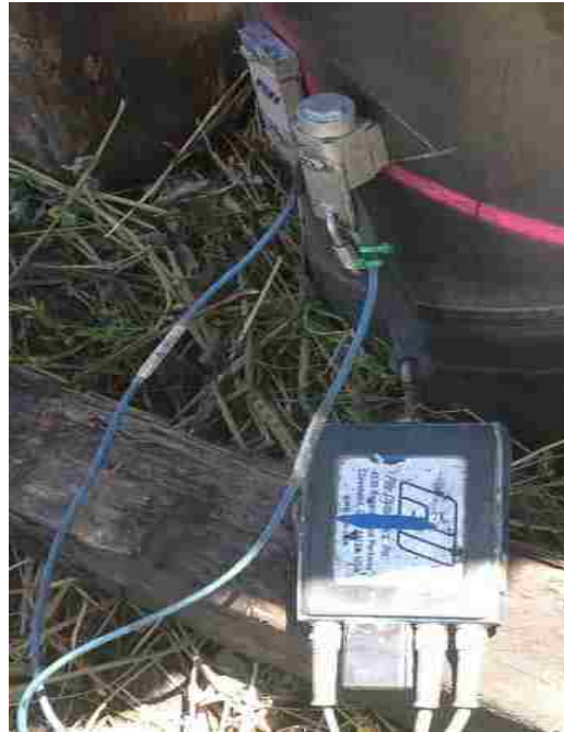
Figure 4.4-1 Accelerometer and strain gauges connected to the top of a pipe pile at the end of driving in connection with PDA measurements.
