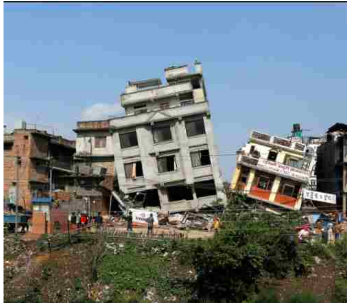
Figure 4-2: Buildings tipped over from differential settlement from the 2015 Kathmandu, Nepal earthquake (after Williams and Lopez, 2015).
