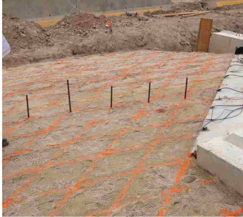
Figure 3-15: Photo of Painted Grid on the Ground Surface to Define Heave
