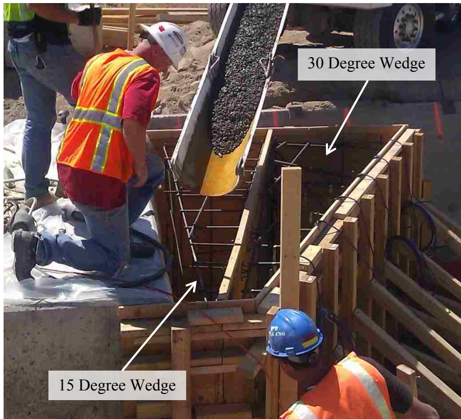
Figure 3-7. Simultaneous casting of 15° and 30° wedges, taken from Marsh (2013).
