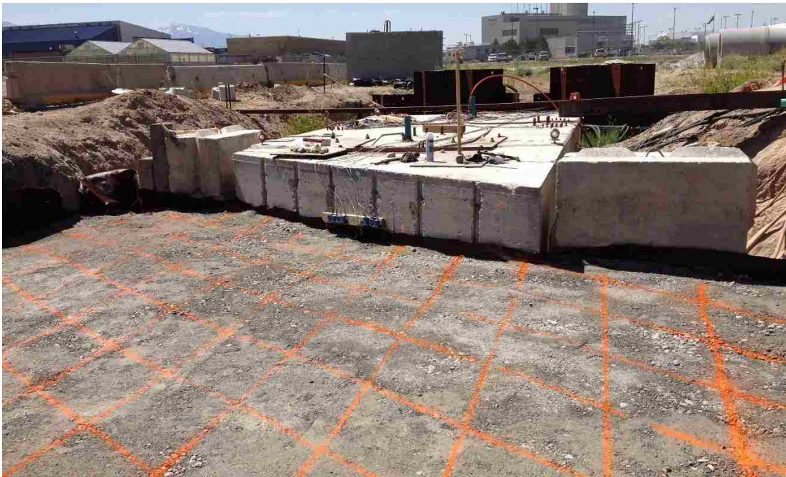
Figure 3-16. Grid painted at 2 ft by 2 ft (0.61 m by 0.61 m) spacing prior to 30° skew GRS test.
