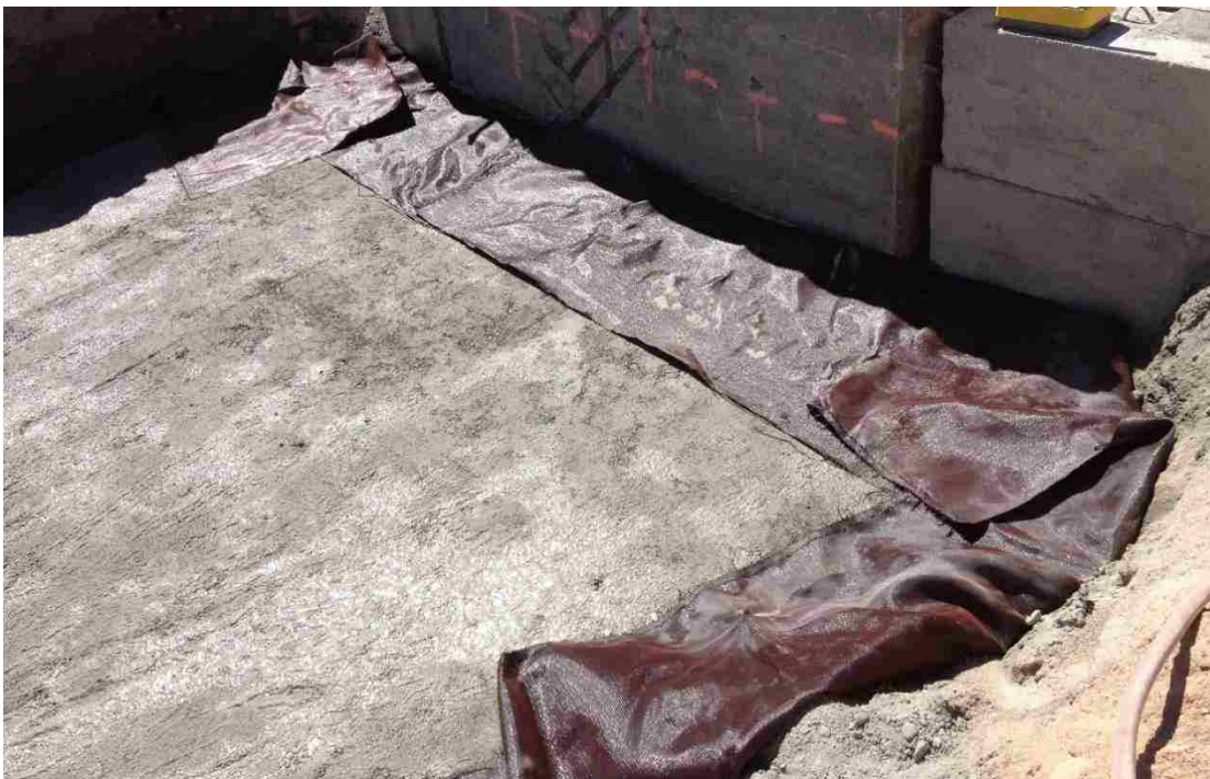
Figure 3-13. Extra geofabric was folded over the 1-ft (0.30-m) gravel layer in the non-skewed GRS test before placement of the next fabric sheet.
