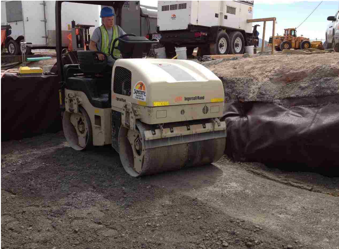
Figure 3-11. Vibratory roller compactor used for the bulk of the gravel compaction.
