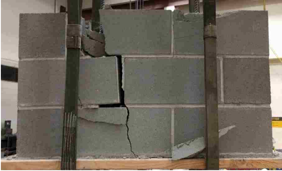
Figure 4-7: Typical Masonry Panel After Failure
