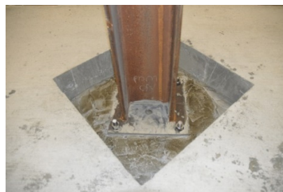
Figure 1-1: Blockout connection commonly used at the base of steel buildings: (a) detail; (b) picture of blockout just after column installation and prior to pouring of blockout concrete.
