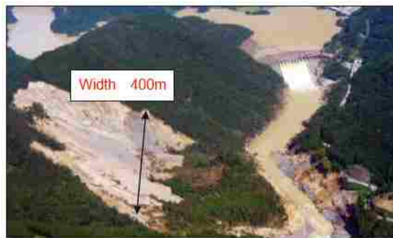
Figure 3-4: Slope failure downstream of the Tsukabaru Dam (Sumi et al. 2015)
