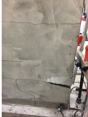
(b) Toe crushing.
