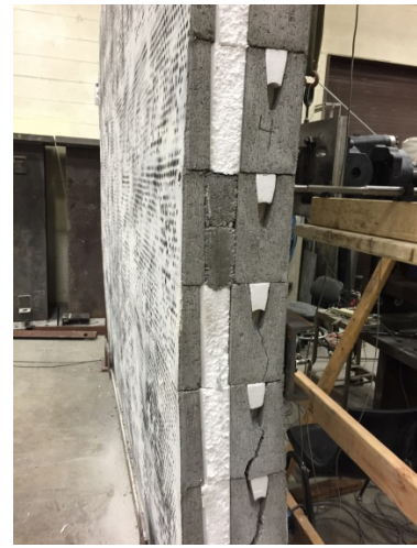
(c) Cracking through webs.
