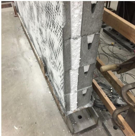
(a) No cracking in webs.
