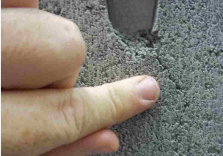
Figure 4-7 Cracking in web prior to testing.
