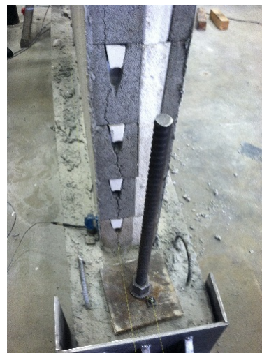
(c) Cracking in webs.
