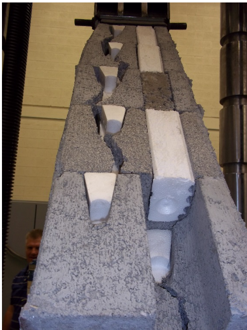
(a) Crack through webs.
