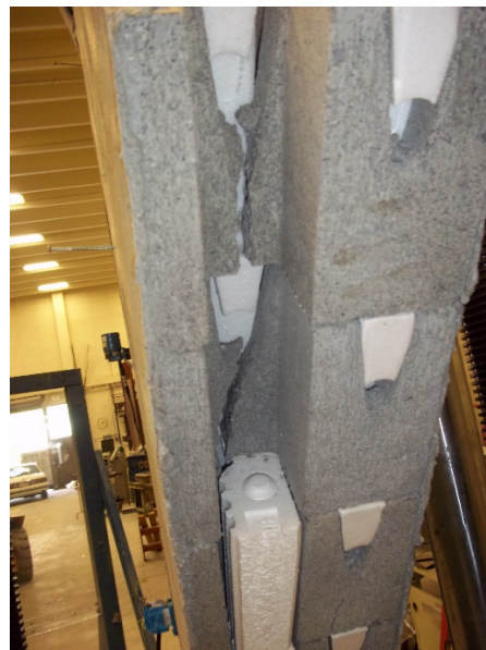
(b) Cracking through webs.
