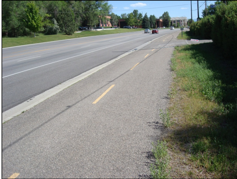
Figure 5-29: Southbound view of the shared use path on University Avenue at Marrcrest East, Provo (photo taken by Chris Haskell, 2015).
