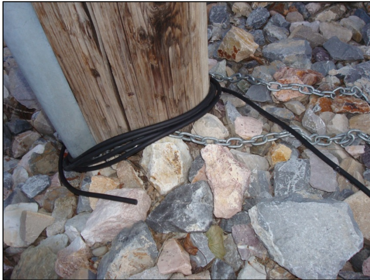
Figure 4-4: Placement of remaining mini tubes (photo taken by Chris Haskell, 2015).
