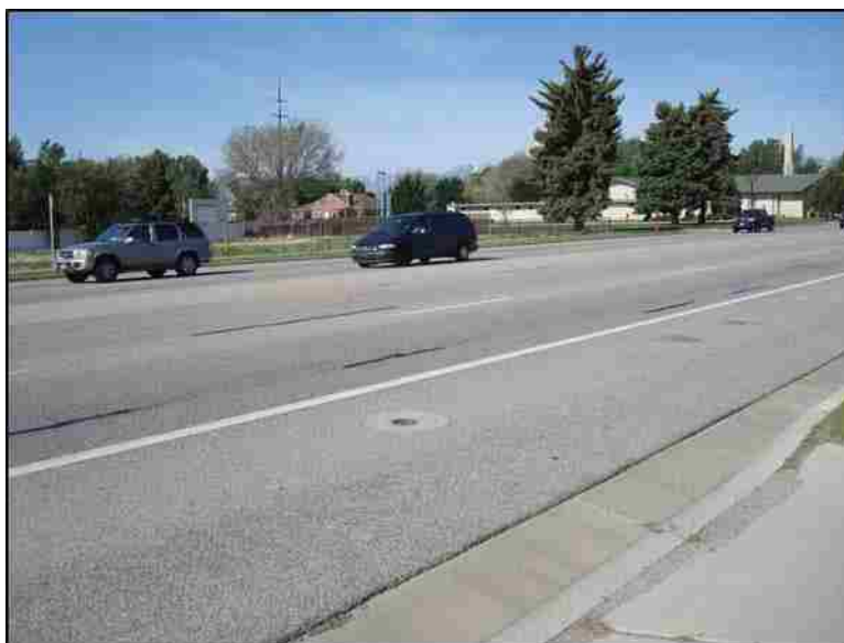
Figure 5-15: View of 10600 South at 1450 West, South Jordan (photo taken by Chris Haskell, 2015).
