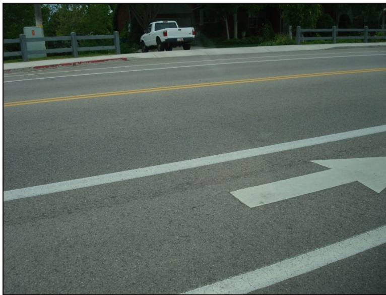
Figure 5-23: View of 800 South at 482 West, Orem (photo taken by Chris Haskell, 2015).
