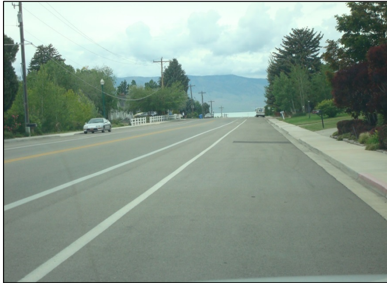
Figure 5-24: Westbound view of the bike lane on 800 South at 482 West, Orem (photo taken by Chris Haskell, 2015).
