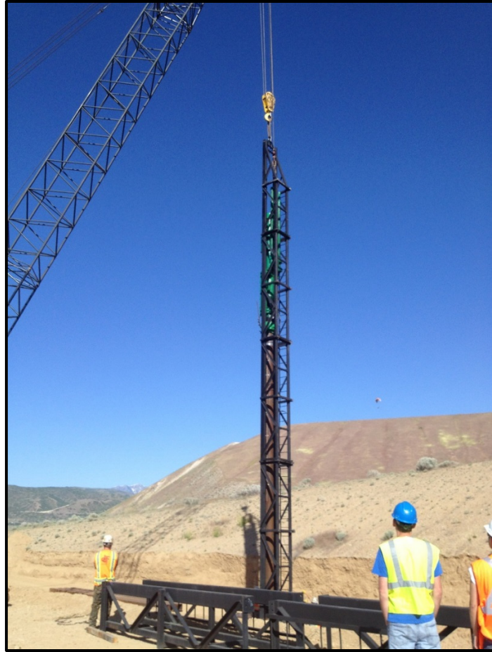
Figure 3-3: Installation of piles using a diesel hammer.
