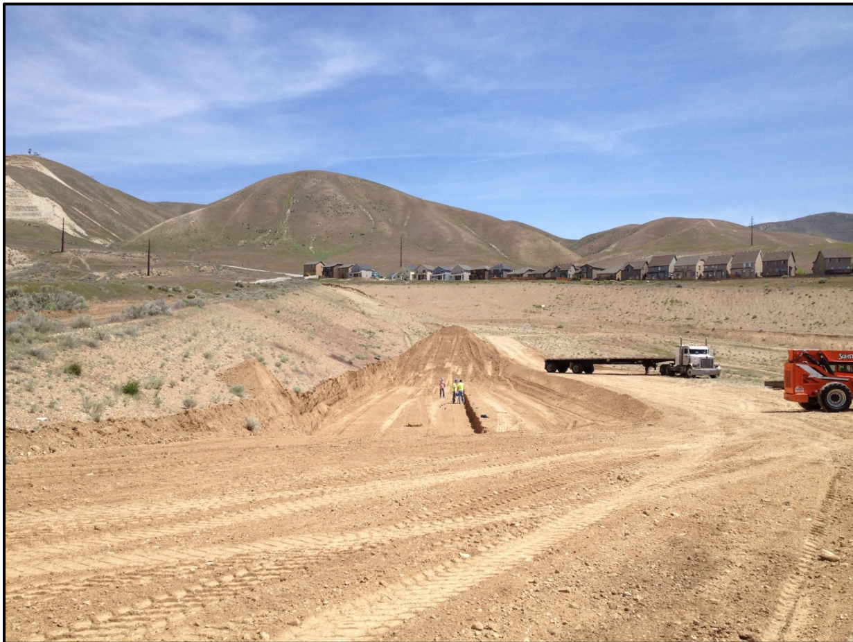
Figure 3-2: Project site after completion of site grading.
