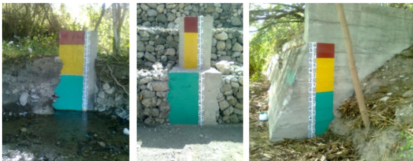
Figure 3-4: Example of staff gauges in Rio Tabara, Rio Grande and Arroyo Grande in the Azua province, Dominican Republic
