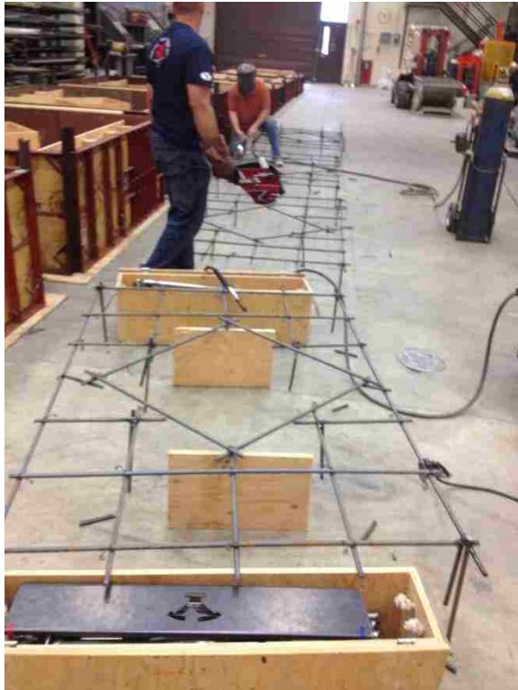
Figure 3-13: Welding on Rebar Chairs
