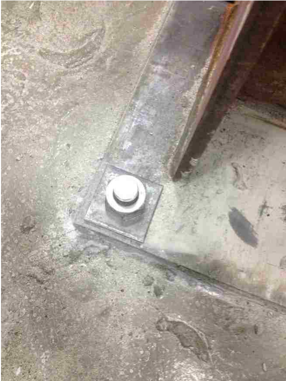
Figure 3-18: Bolt and Washer Installed on Grouted Column
