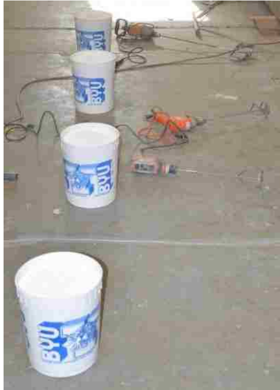
Figure 3-24: HYDROCAL Mix Preparation
