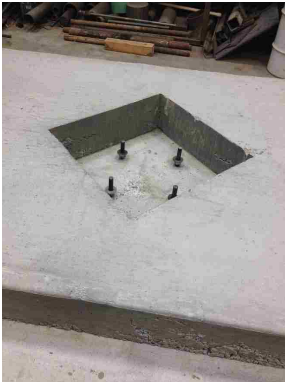
Figure 3-16: Leveling Nuts and Washers
