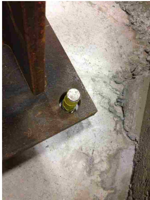
Figure 3-17: Column on Leveling Nuts and Washers
