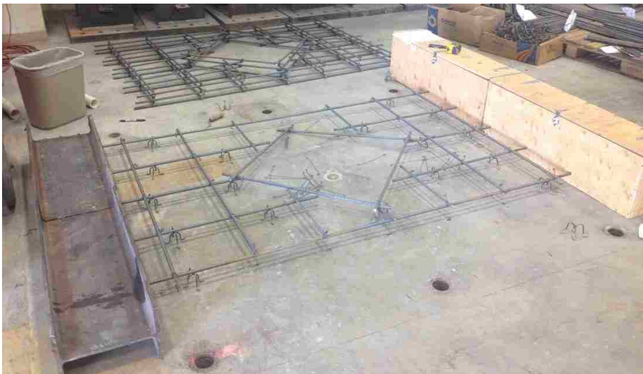
Figure 3-6: Tying the Slab Rebar
