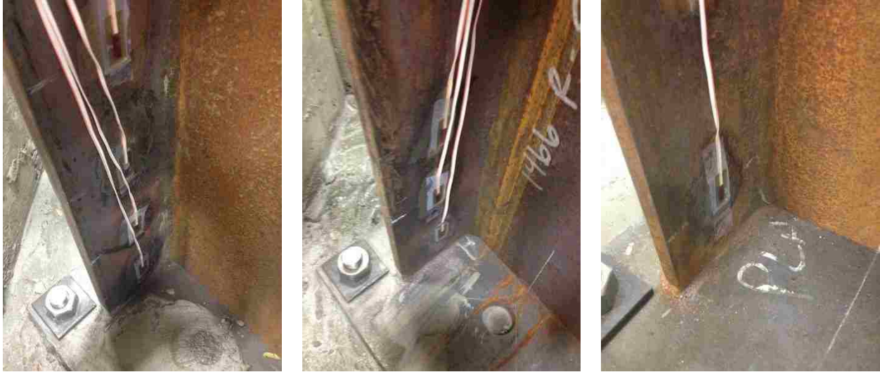
Figure 3-31: Installed Strain Gages
