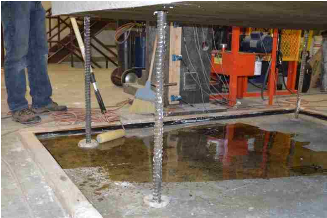
Figure 3-23: Applying Form Release to Lab Floor
