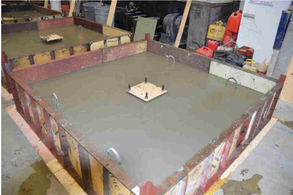
Figure 3-11: Completed Footing
