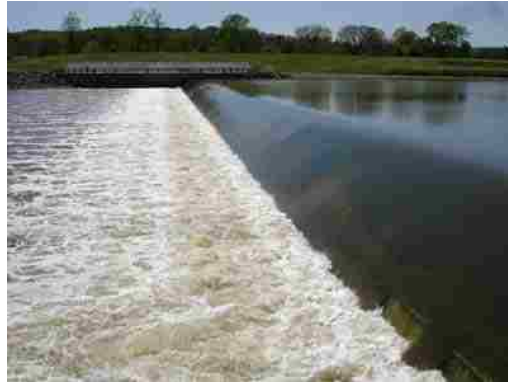
Figure 1: Typical Low-Head Dam, (NIOSH, 2010)
