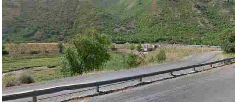
Figure 34. Control Structure in Hobbie Creek
