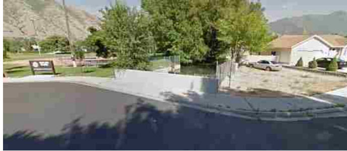
Figure 18. Channeled Section of Hobble Creek in Springville (Source: Google Maps)
