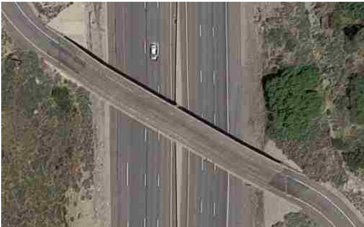
Figure 2-15: A narrow skewed bridge located near utility exit 133 off of Interstate-80, about 5 miles east of Salt Lake City, Utah (adapted from Google Earth)
