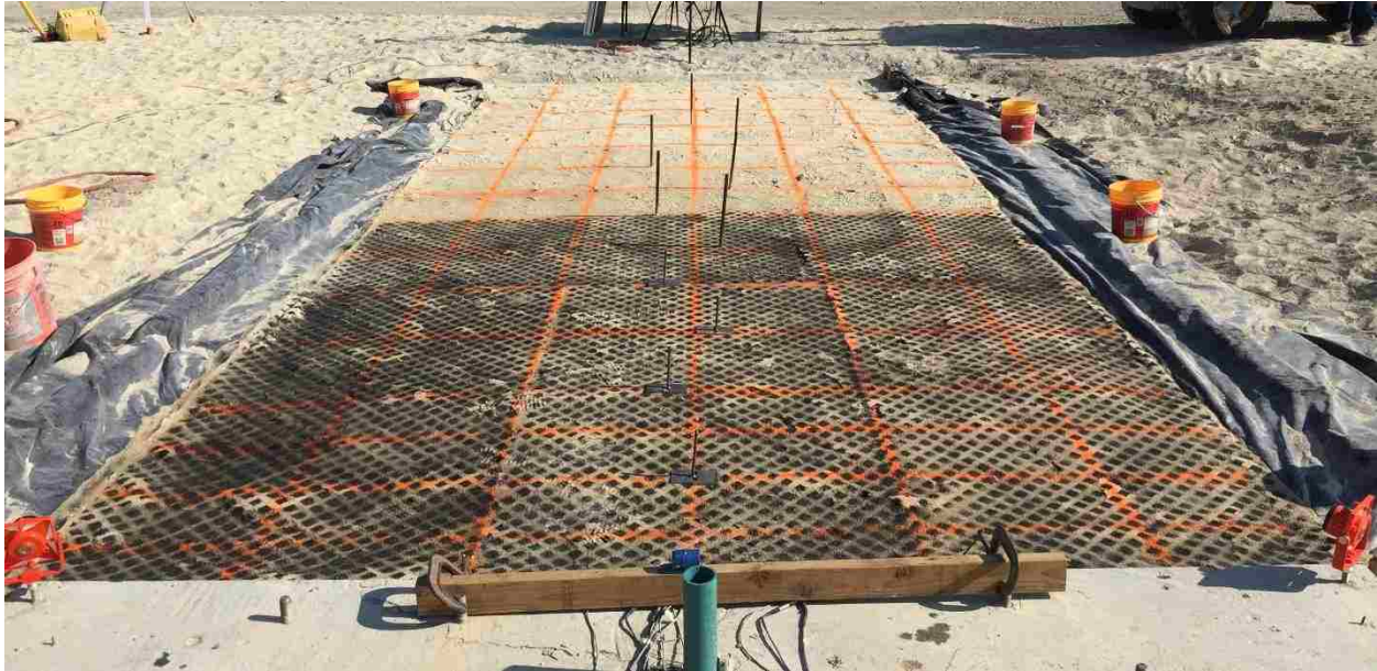
Figure 4-4: Photo of the grid line layout for the 0° skew test
