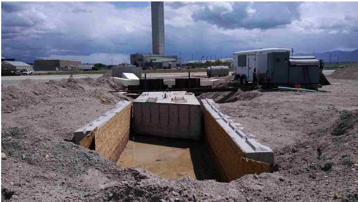
Figure 3-6: Interlocking pre-cast block walls with plywood sheeting
