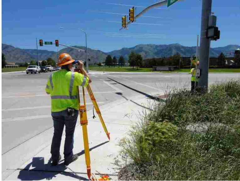
Figure 3-8: Measurement of roadway elevations.
