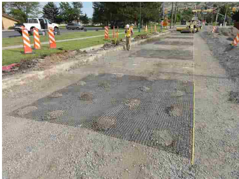
Figure 3-5: Installation of geogrid reinforcement at Orem site.
