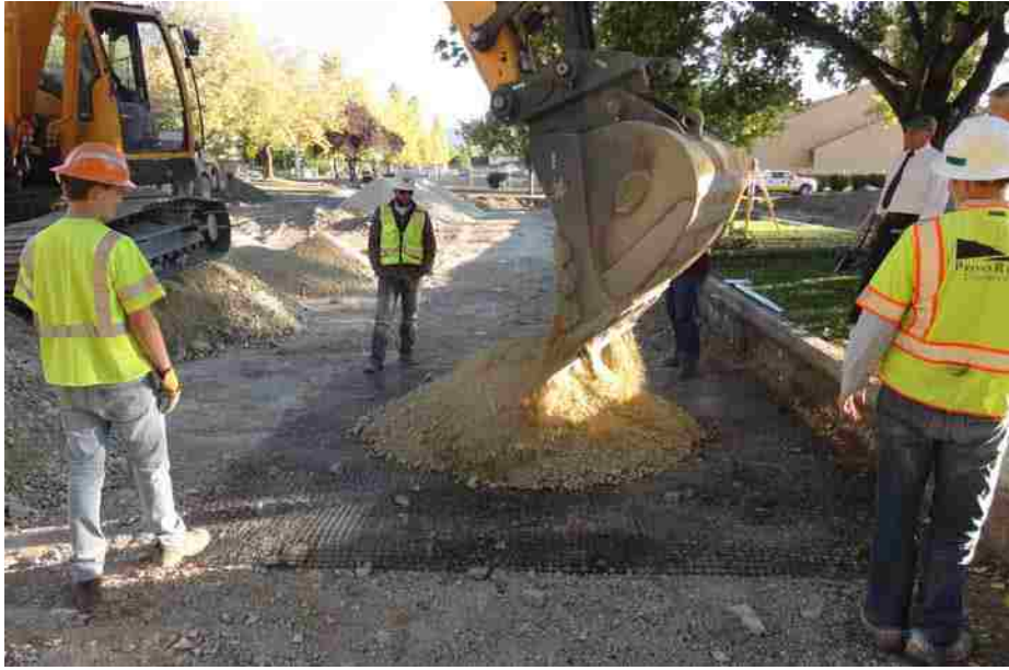
Figure 3-10: Installation of geogrid reinforcement at Springville site.
