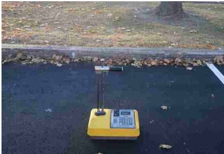
Figure 3-15: NDG testing of HMA layer.
