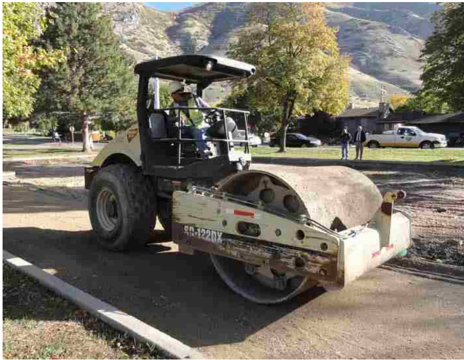
Figure 3-11: Vibratory roller for compaction of base layer at Springville site.
