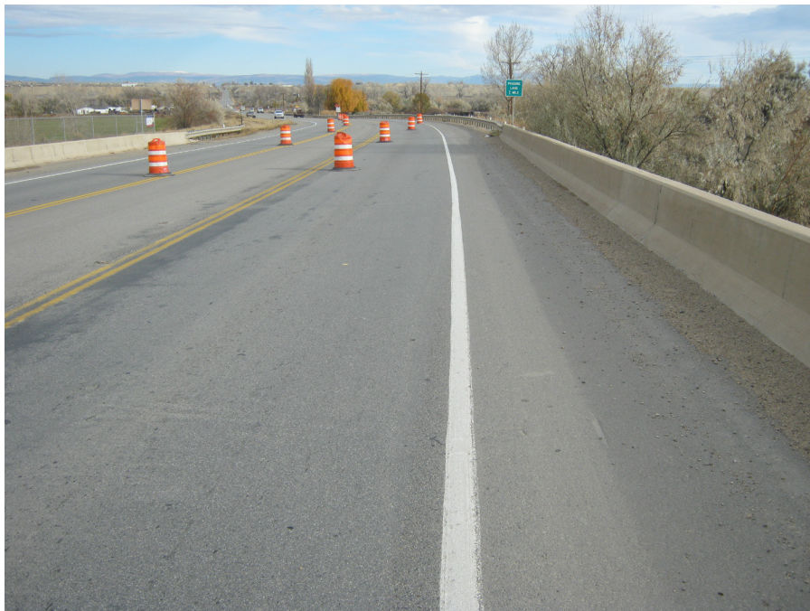
Figure 2-6: Deck with asphalt overlay.
