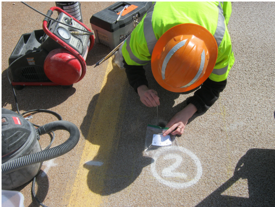
Figure 3-5: Concrete sampling for chloride concentration analysis.
