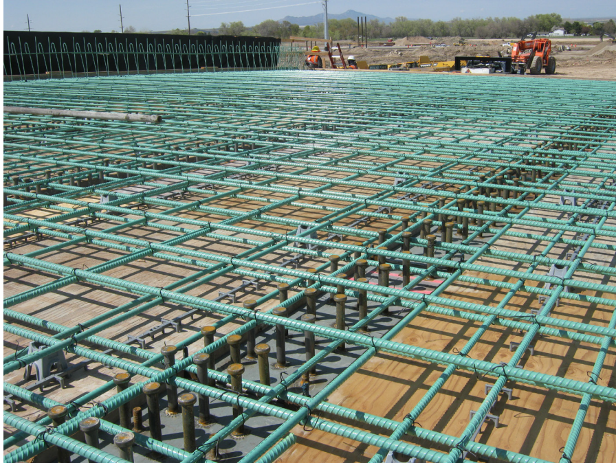
Figure 2-5: Epoxy-coated reinforcement.
