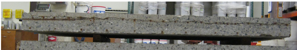
Figure 2-3: Delaminated concrete bridge deck slab.
