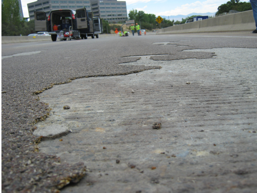
Figure 2-9: Delamination of polymer overlay.
