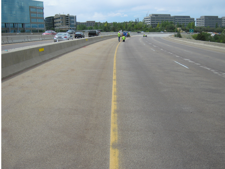
Figure 2-7: Deck with polymer overlay.
