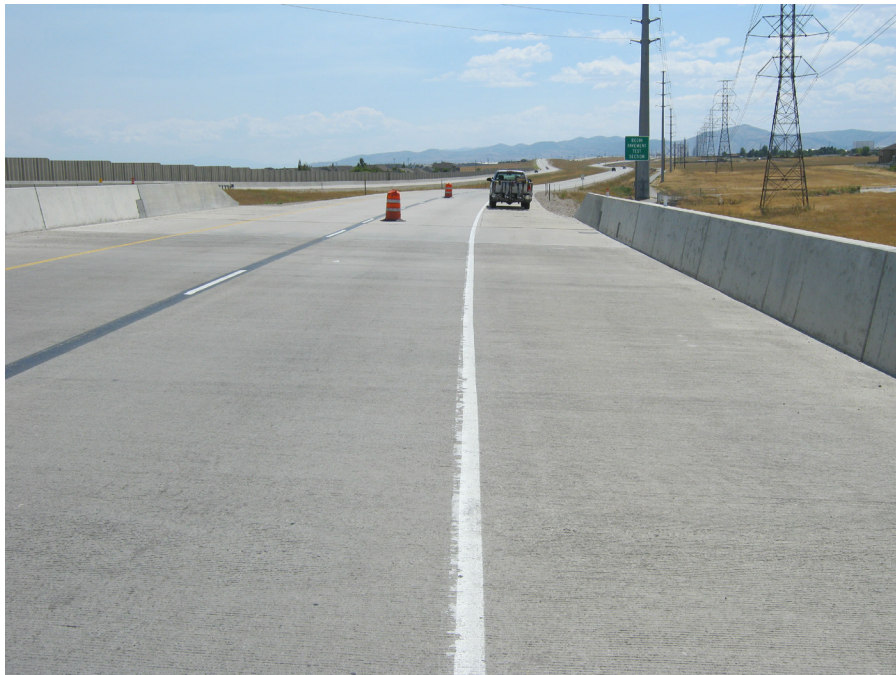
Figure 1-1: Bare concrete bridge deck.
