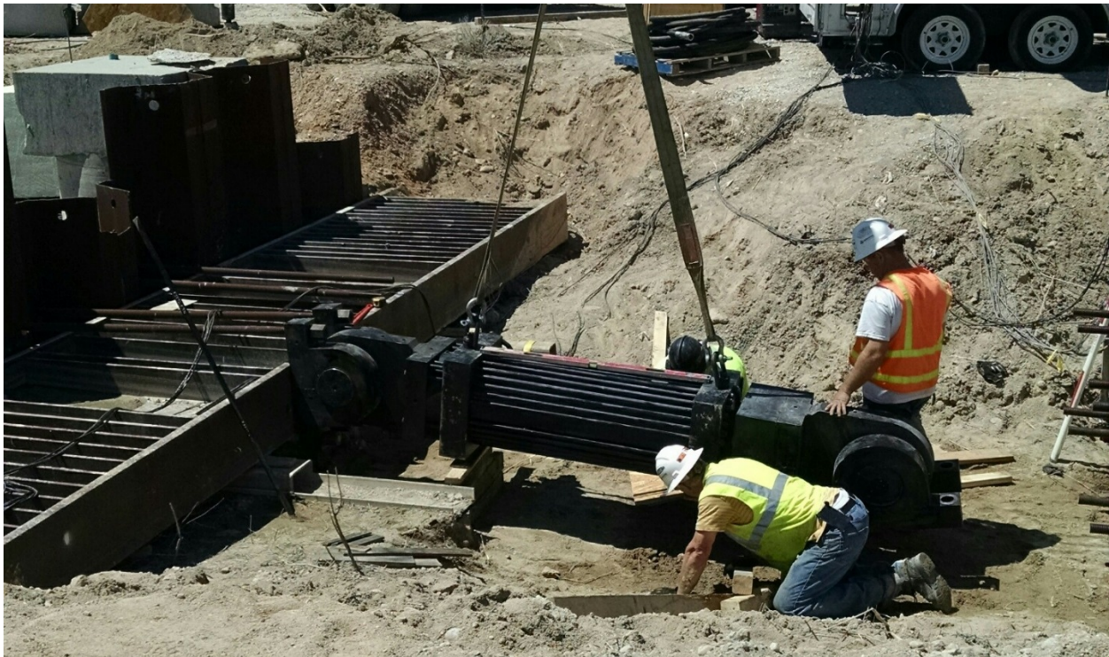
Figure 3-3: Hydraulic actuator placement at Salt Lake Airport test site.
