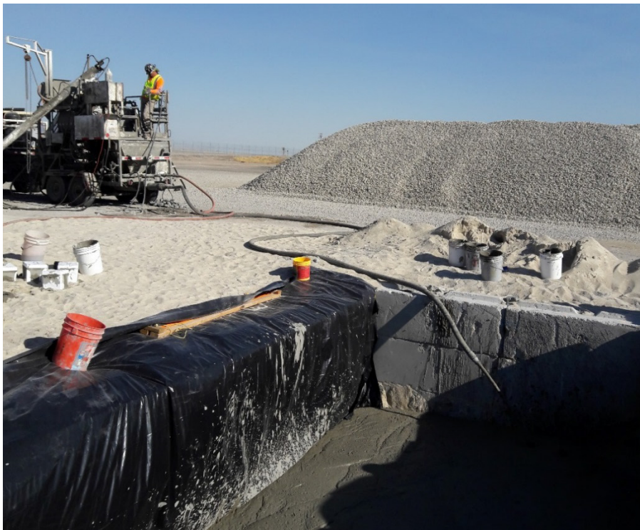
Figure 3-16: Cellular concrete placement by pumping unit for the 0° skew backfill.
