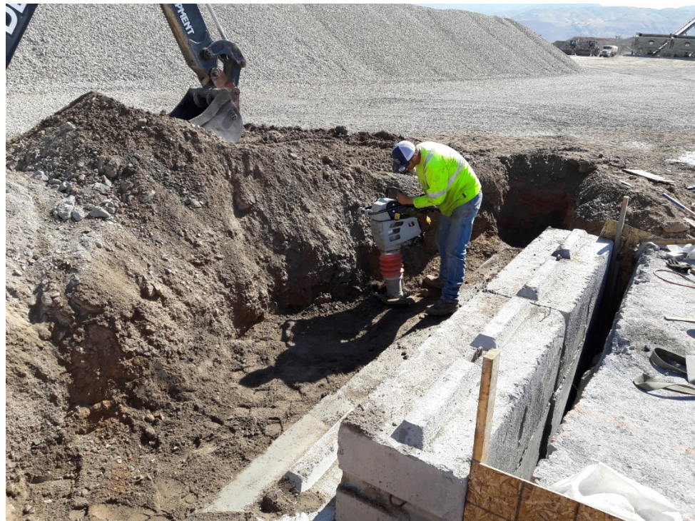
Figure 3-7: Construction of reaction block wall to alter test layout.
