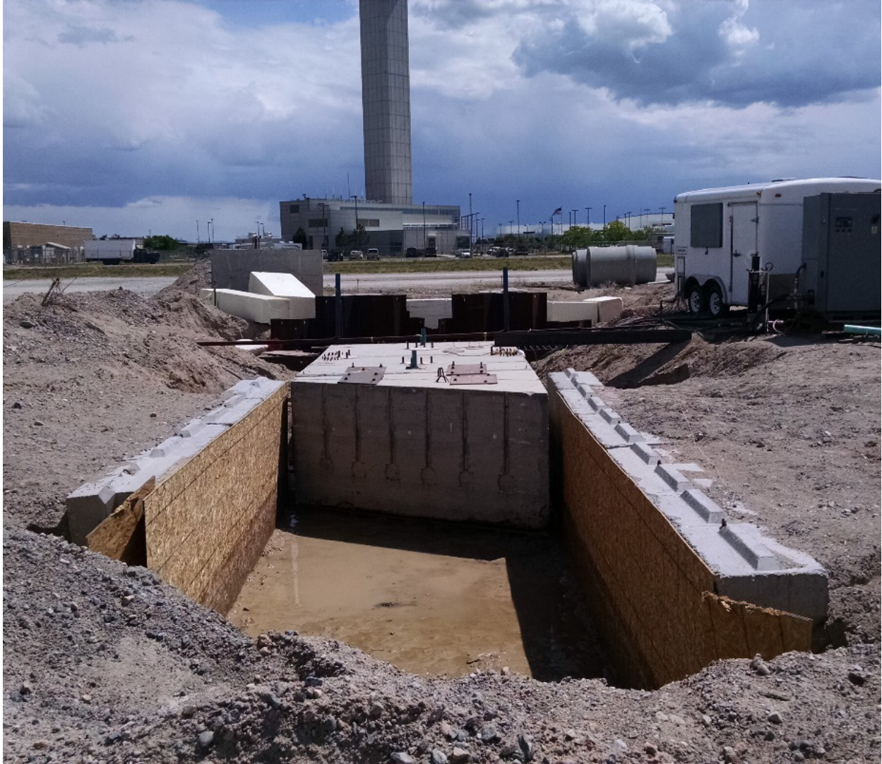
Figure 3-5: Backfill area at Salt Lake Airport test site.
