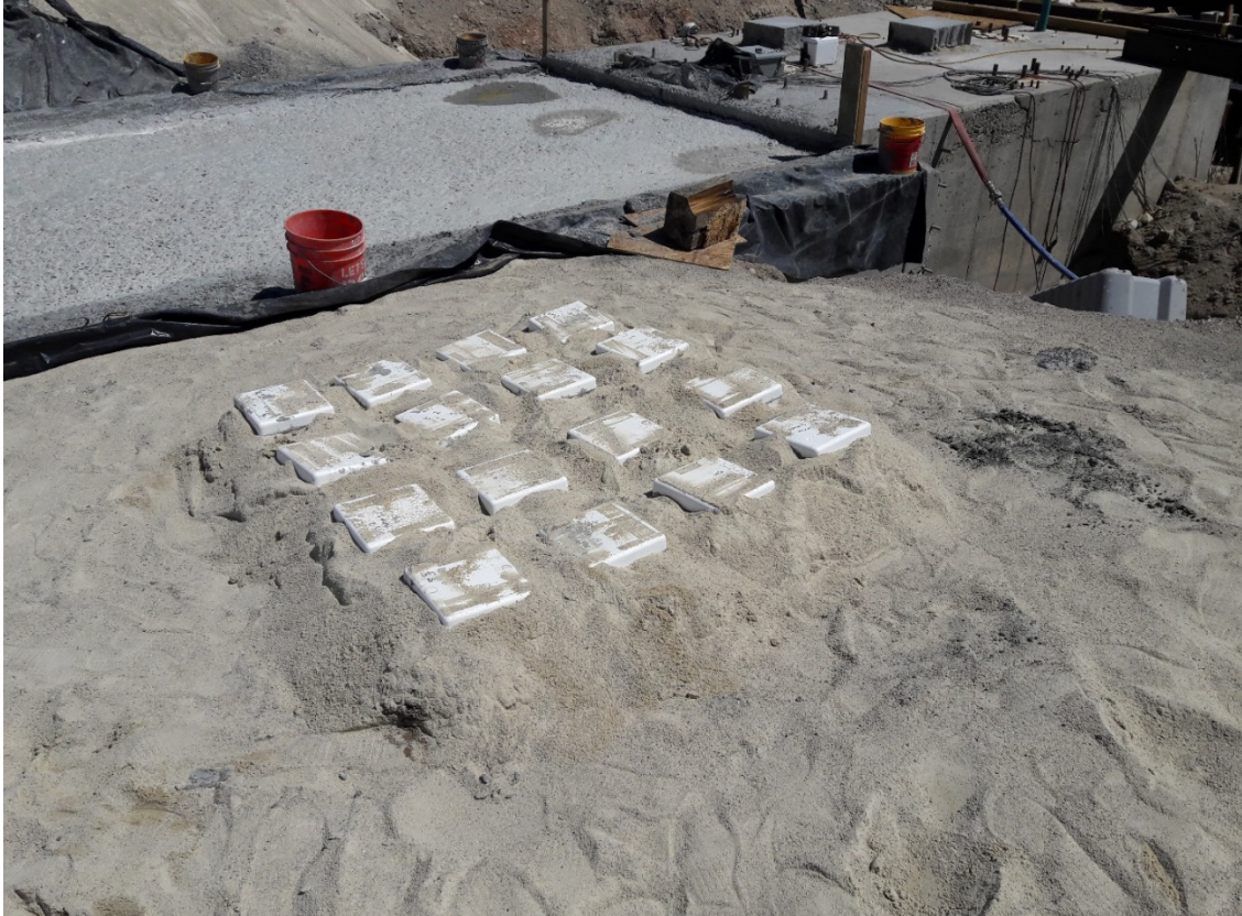
Figure 4-3: Cellular concrete cylinders left to cure on site.
