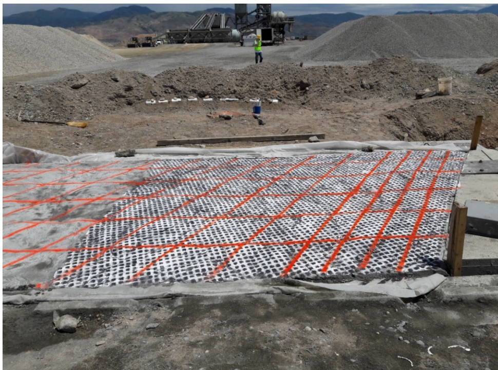
Figure 3-11: 30° skew backfill surface before testing.
