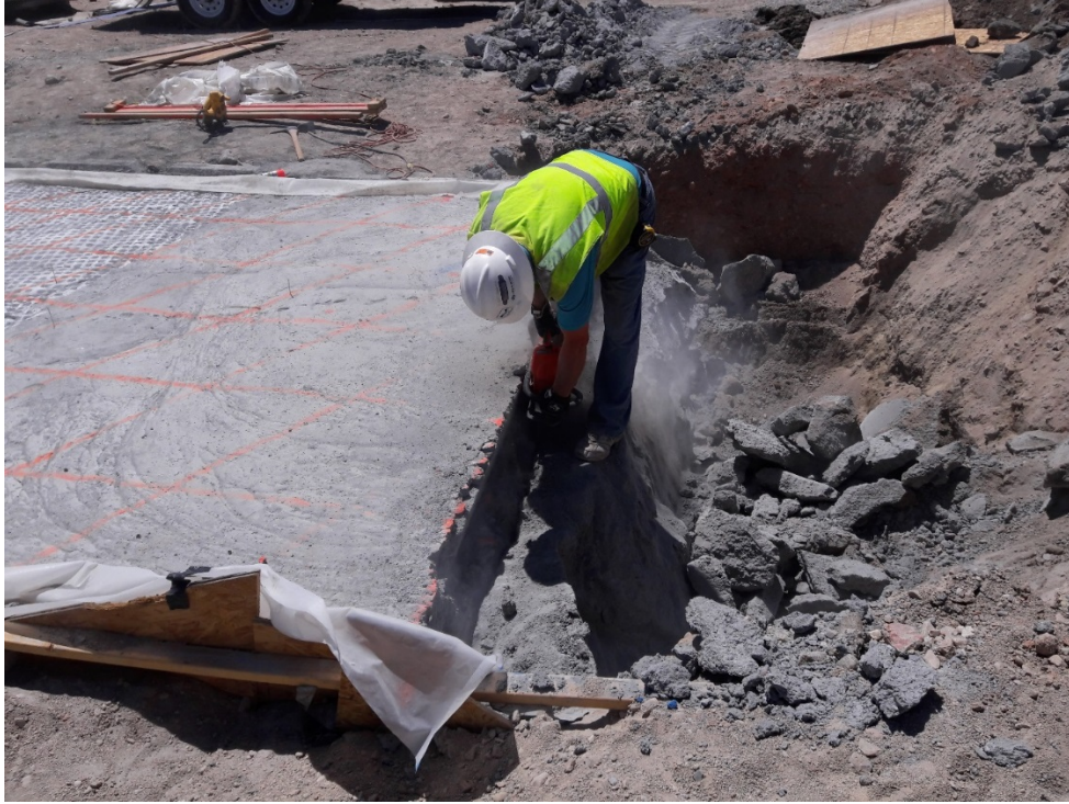
Figure 3-6: Excavation of backfill to alter test layout.
