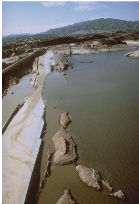
Figure 2-12: Flow Liquefaction of the Lower San Fernando Dam, 1971 (courtesy of NOAA/NGDC, E.V. Leyendecker, U.S. Geological Survey)
