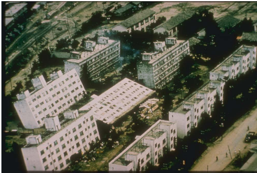
Figure 2-13: Bearing Capacity Failure from Soil Liquefaction During the Niigata, Japan (1964) Earthquake (courtesy of NOAA/NGDC – National Geophysical Data Center)
