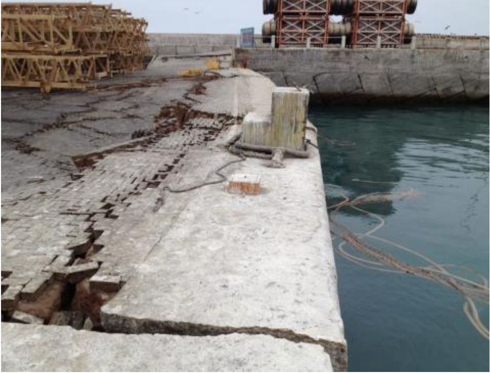
Figure 2-11: Lateral Displacement Near the End of the Molo Pier after the Iquique (Chile), 2014 Earthquake (after GEER, 2014)
