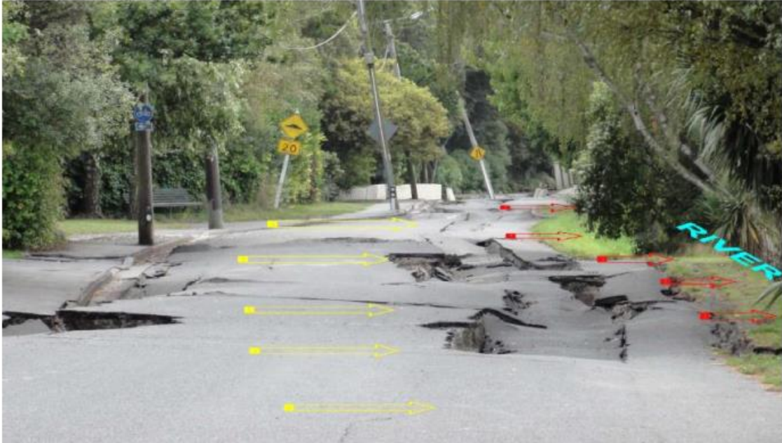
Figure 2-10: Example of Lateral Spreading along the Avon River after the Christchurch, 2011 Event (after GEER, 2011)
