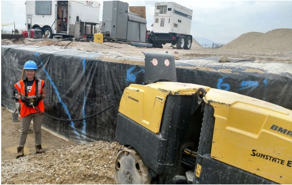
Figure 3-11. Rebecca Black operating a trench compactor.
