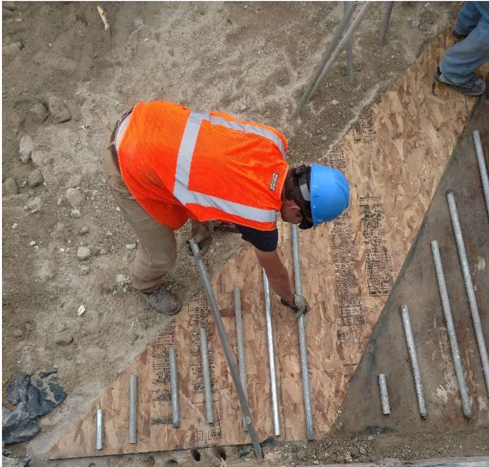
Figure 3-7. Galvanized steel pipe rollers being installed on completed skew wedge bases.
