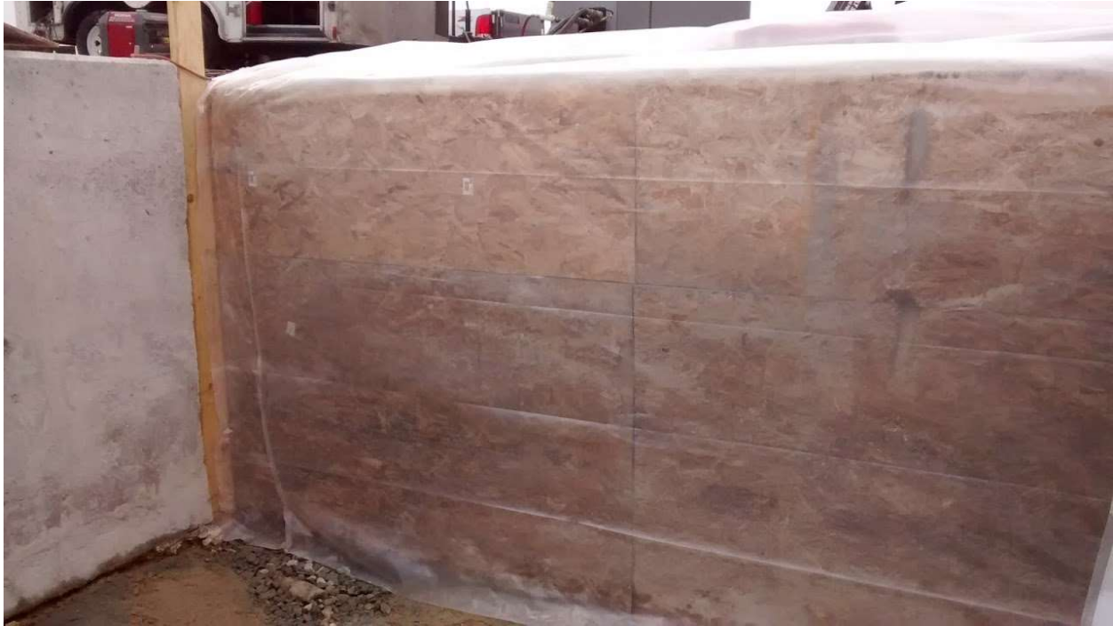
Figure 3-5. Box side wall covered with plywood and first layer of plastic.
