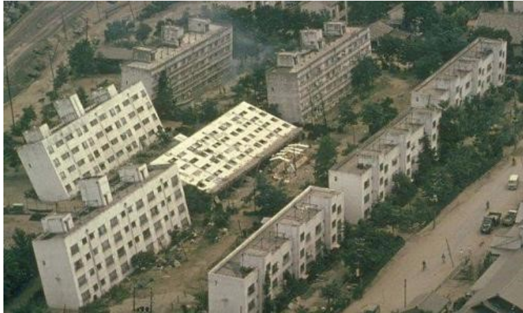
Figure 3-21: Example of a loss of bearing capacity failure causing apartment buildings to collapse in Niigata, Japan, after the 1964 earthquake (after Kramer (1996)).
