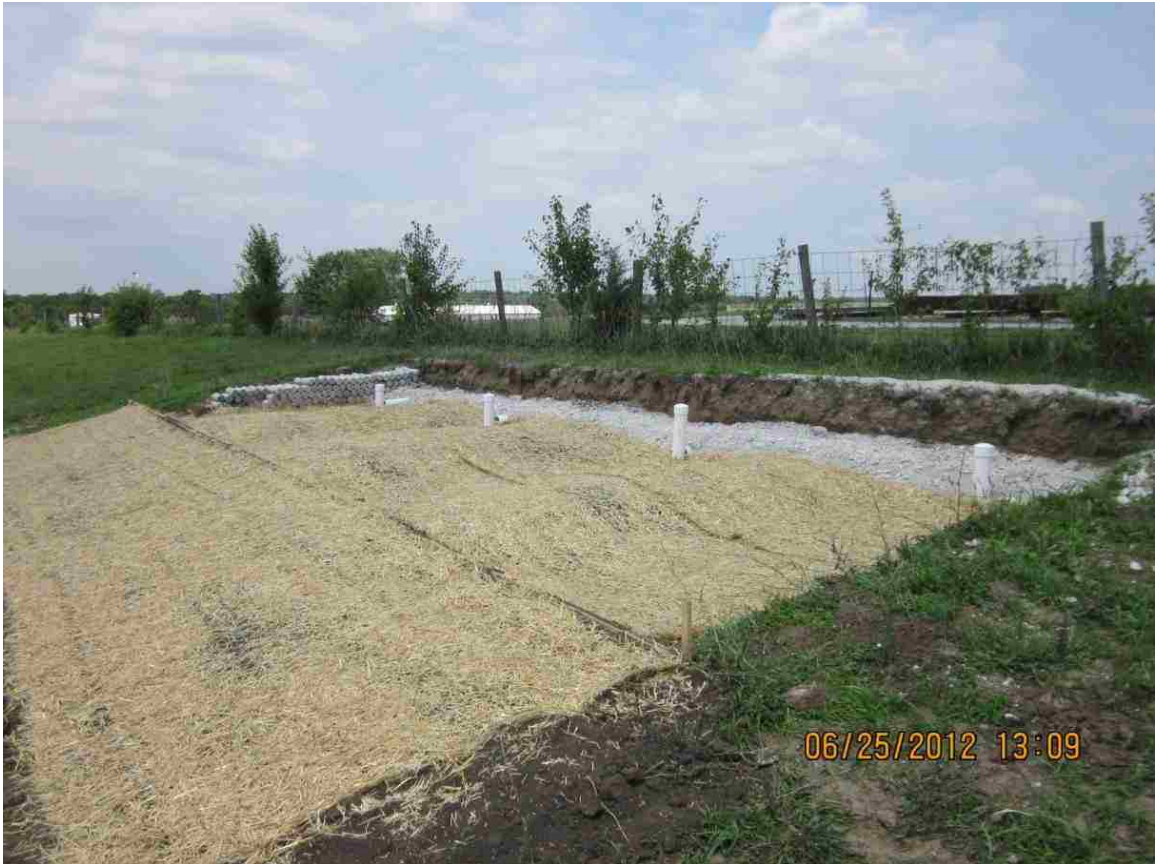
Figure B.1 Bioretention after construction
