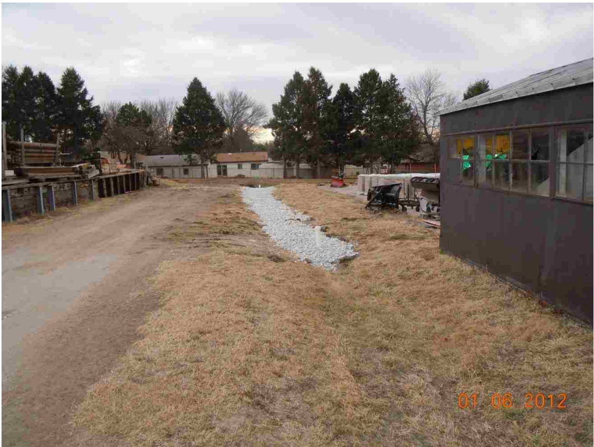
Figure B.5 Infiltration trench after construction
