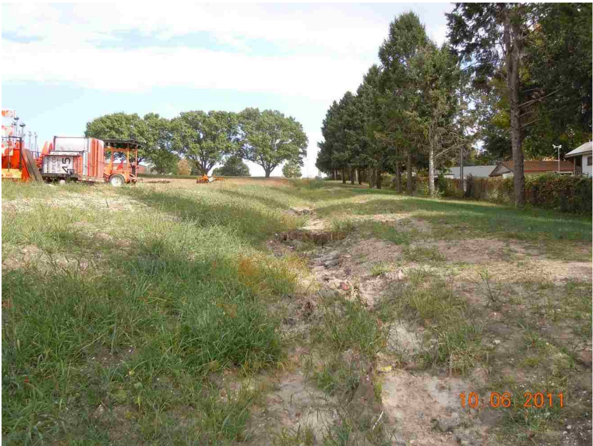
Figure B.6 Filter trench before construction
