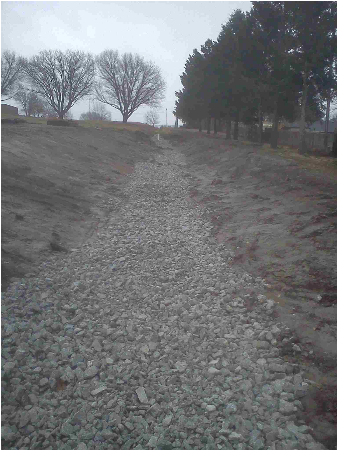
Figure B.7 Filter trench after construction
