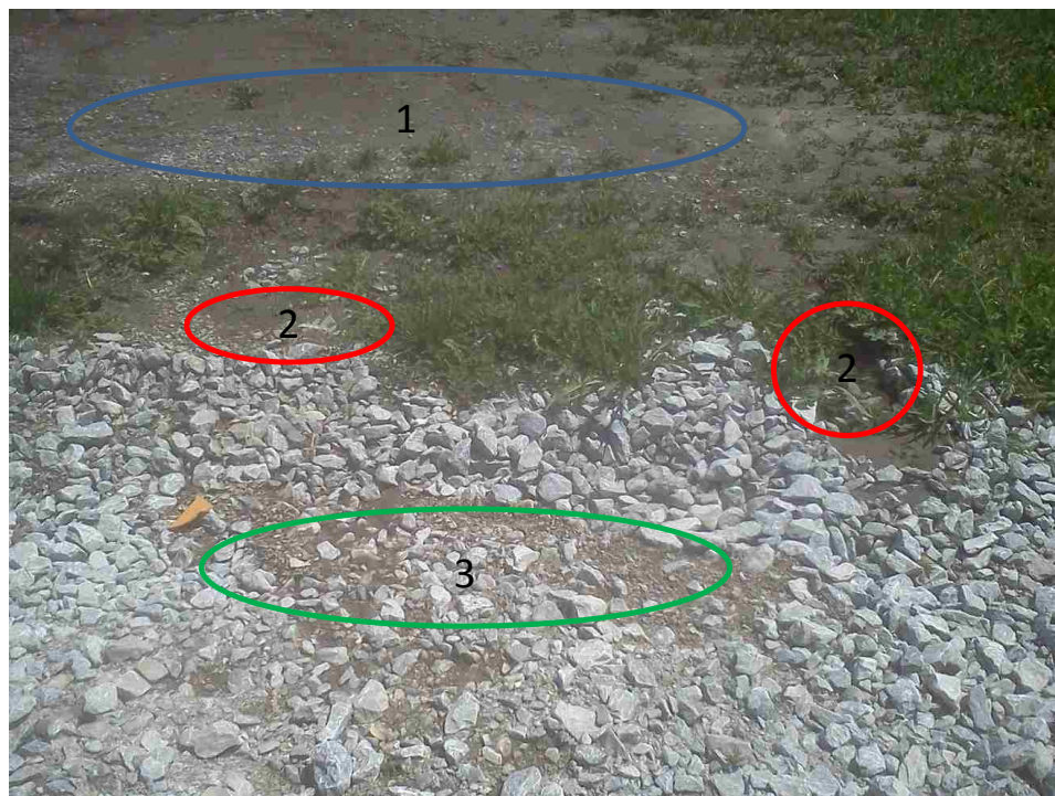
Figure 2.19 Infiltration trench clogging
