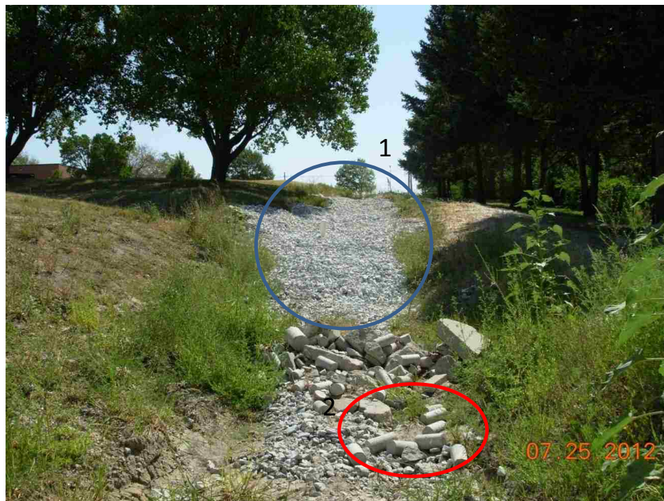
Figure 2.24 Filter trench added 1-3 inch rock at beginning and check dam material migration (water flow direction: from the top to bottom of the picture)
