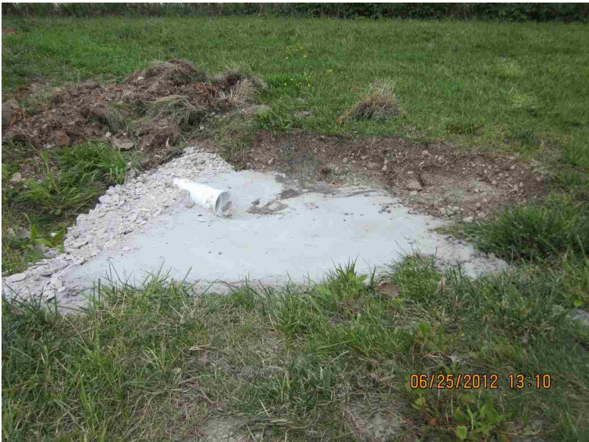
Figure B.9 Bioretention diversion after construction
