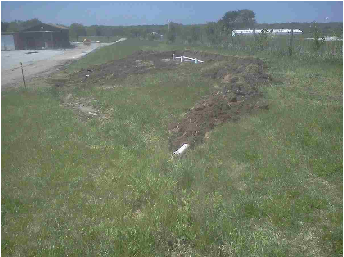
Figure B.8 Bioretention diversion during construction
