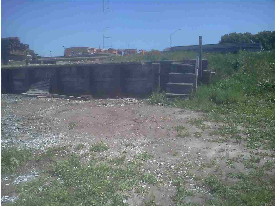
Figure B.10 Small disturbed area by infiltration trench
