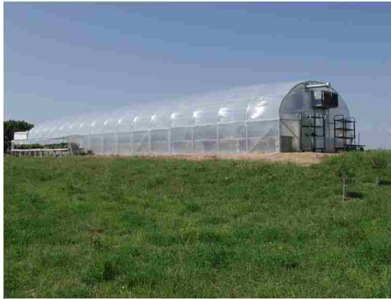
Figure 1.3. Quonset Style Greenhouse at Firth NE (West Side).
