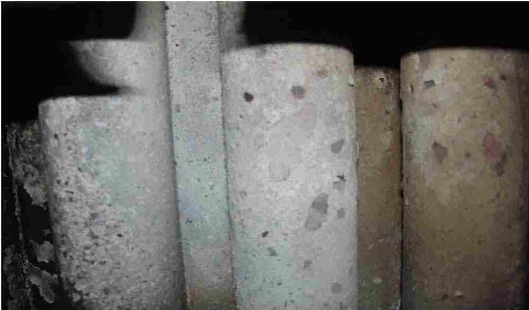
Figure 3.7. Fouling of Heat Exchanger Pipes.
