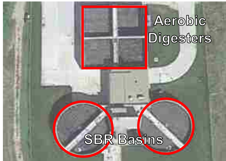
Figure 2.6: Aerial View of a Typical SBR Plant (Google Maps, 2017c).
