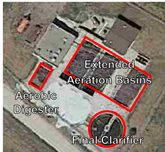
Figure 2.2: Aerial View of a Typical Extended Aeration Plant (Google Maps, 2017a).
