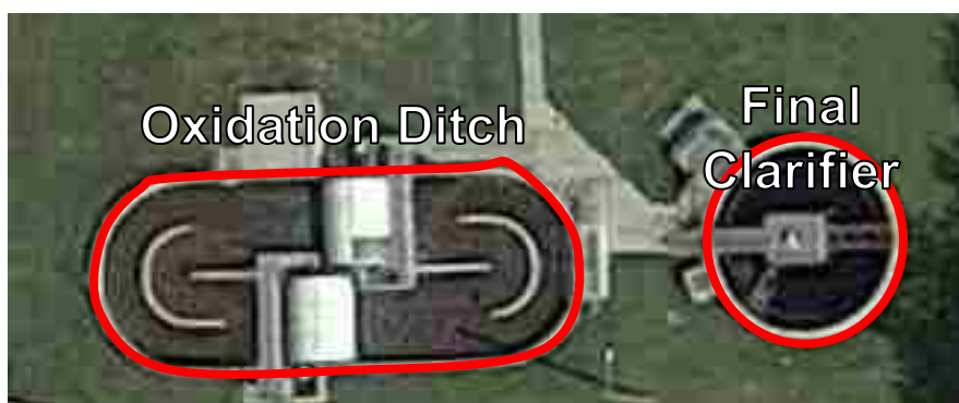
Figure 2.4: Aerial View of a Small Oxidation Ditch Plant (Google Maps, 2017b).
