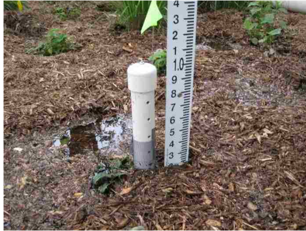
Figure 14. Staff gage and stilling well which houses the pressure transducer.
