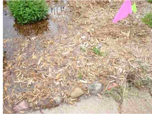
Figure 42. Inundated garden showing widespread outflow onto driveway (designed outflow structure is on opposite side of garden).
