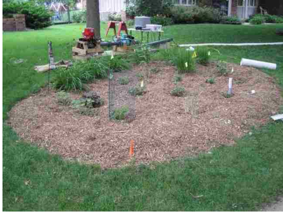
Figure 29. View of rain garden with valve and meter delivery system in background. Note white stilling well is installed at surveyed low-point.
