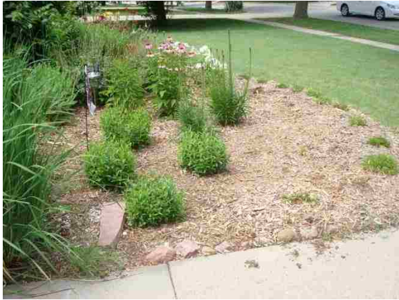
Figure 41. Rain garden constructed against residential foundation (out of picture left). Downspout empties just left of large flagstone piece.
