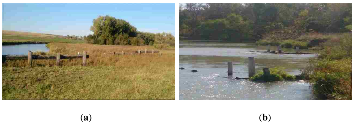
Figure 2.3 Jetties installed in 1950 at Site 5 (a) and in 2000 at Site 4 (b). Note the sediment that has accumulated over time in front of the jetties installed in 1950.
