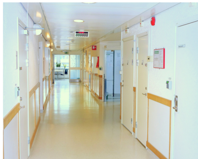
Fig. 10. Portion of a ward in Control hospital showing the corridor-based floor layout that prevented observation from a central point or seating and activity spaces accessed from the corridor.
