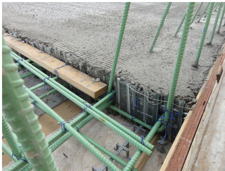
Figure 3-11 Metal shoring used in deck construction process.
