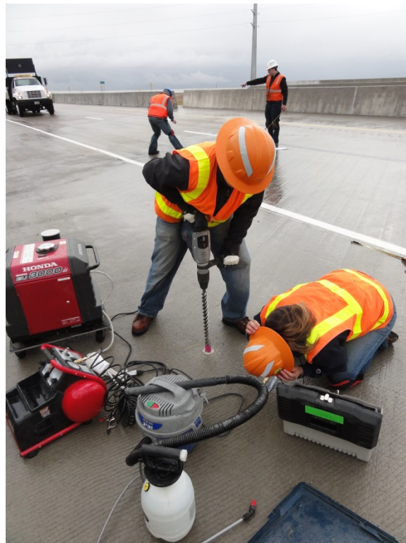
Figure 3-19 Concrete sampling for chloride concentration testing.
