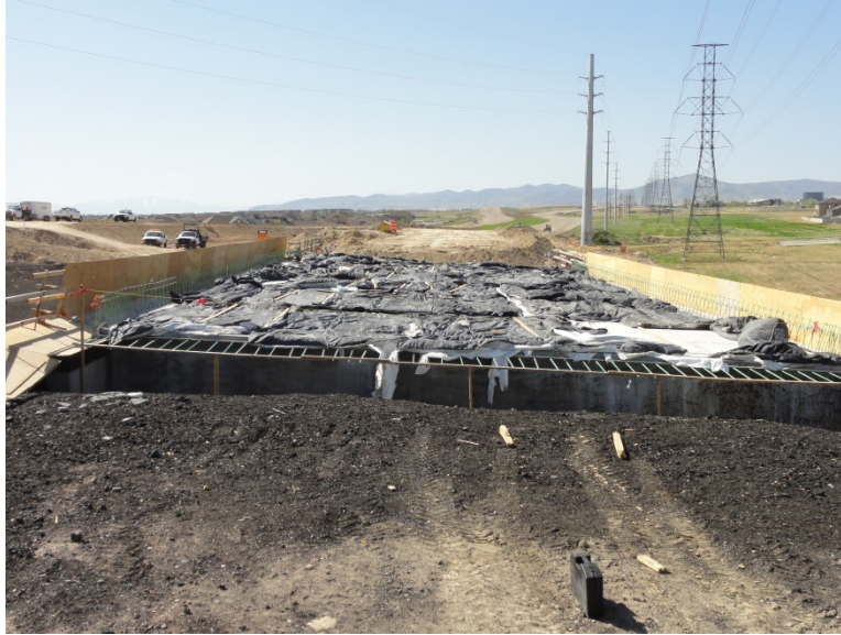
Figure 3-12 Covered bridge deck during curing.
