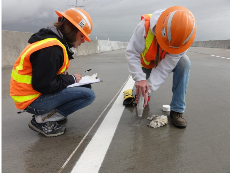
Figure 3-16 Schmidt rebound hammer testing.
