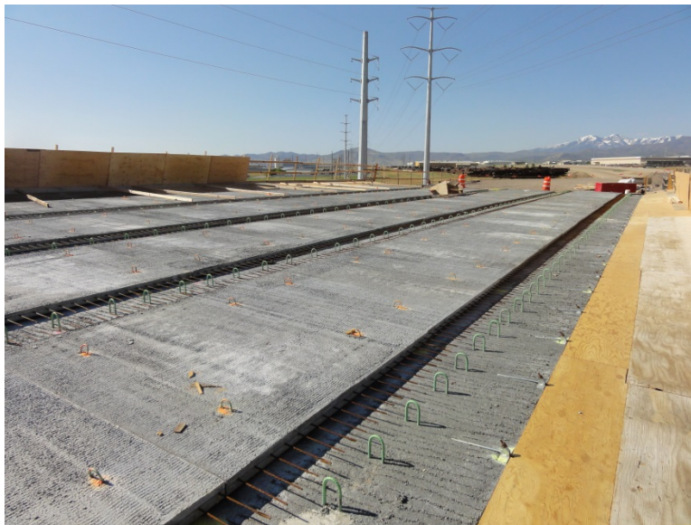
Figure 3-5 Half-deck concrete panels.
