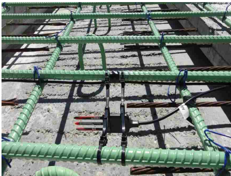
Figure 3-6 Sensor installed at level of top mat of reinforcement.
