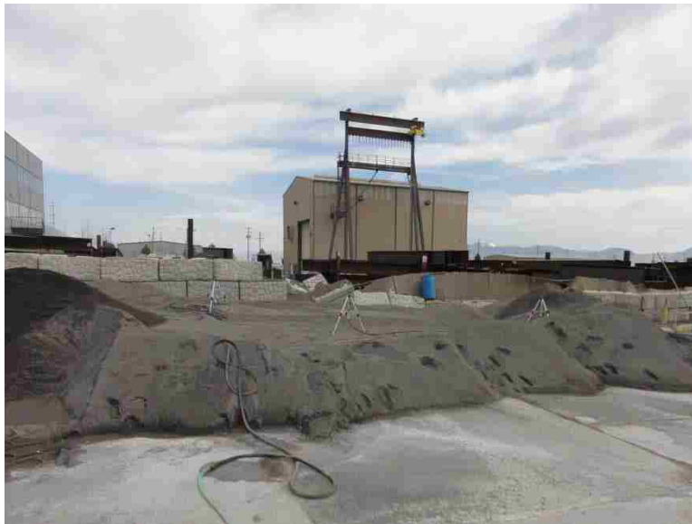
Figure 3-10 Pre-wetting of lightweight fine aggregate at concrete batch plant.
