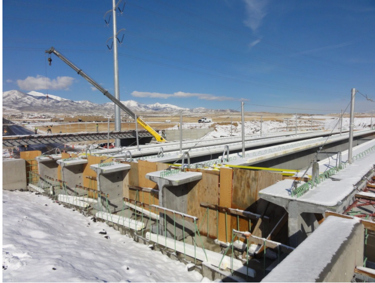
Figure 3-2 Pre-stressed, pre-cast, single-span concrete girders.
