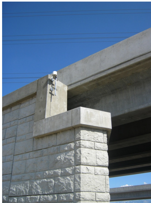
Figure 3-9 Precipitation gauge mounted on bridge.
