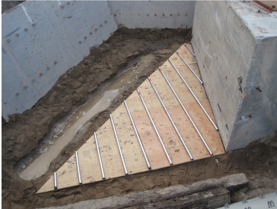
Figure 3.7. Rollers underneath 45° skew wedge.
