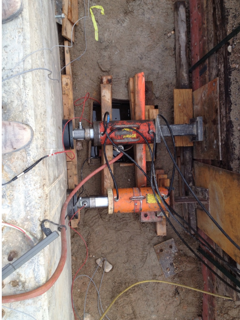
Figure 3.22. 300-kip hydraulic jacks.
