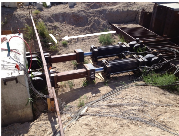
Figure 3.18. 600-kip hydraulic actuators.
