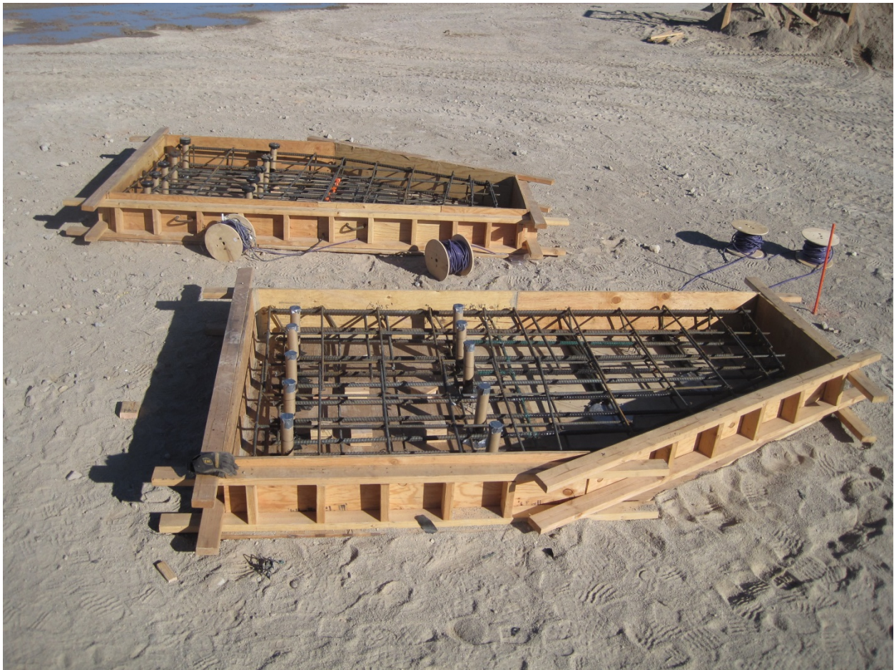
Figure 3.15. Wingwall reinforcement cages and forms.
