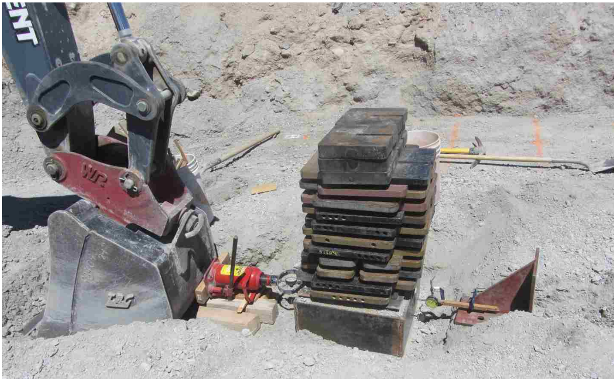
Figure 3.31. In-situ direct shear test setup.
