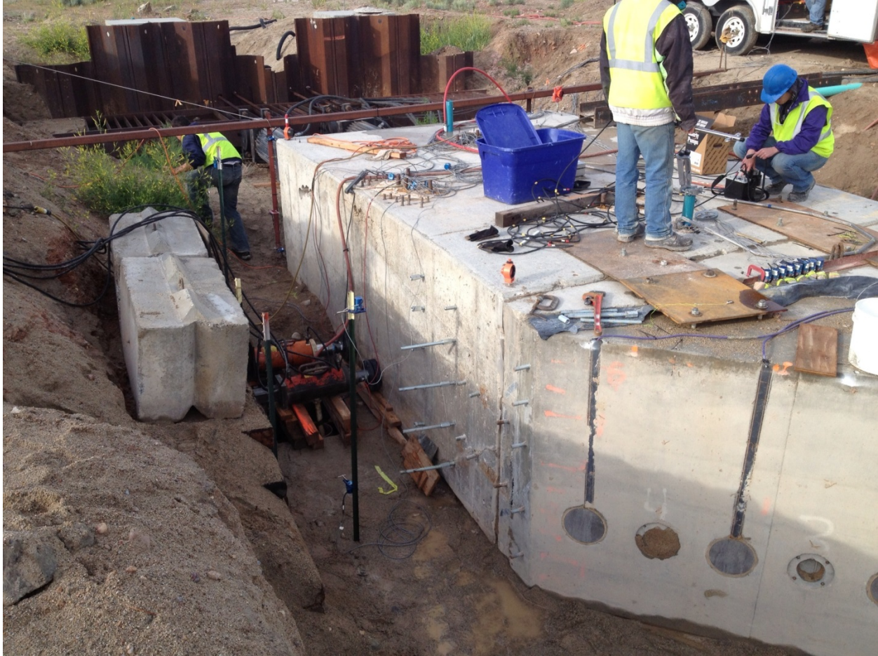
Figure 3.21. Transverse load-deflection test setup.
