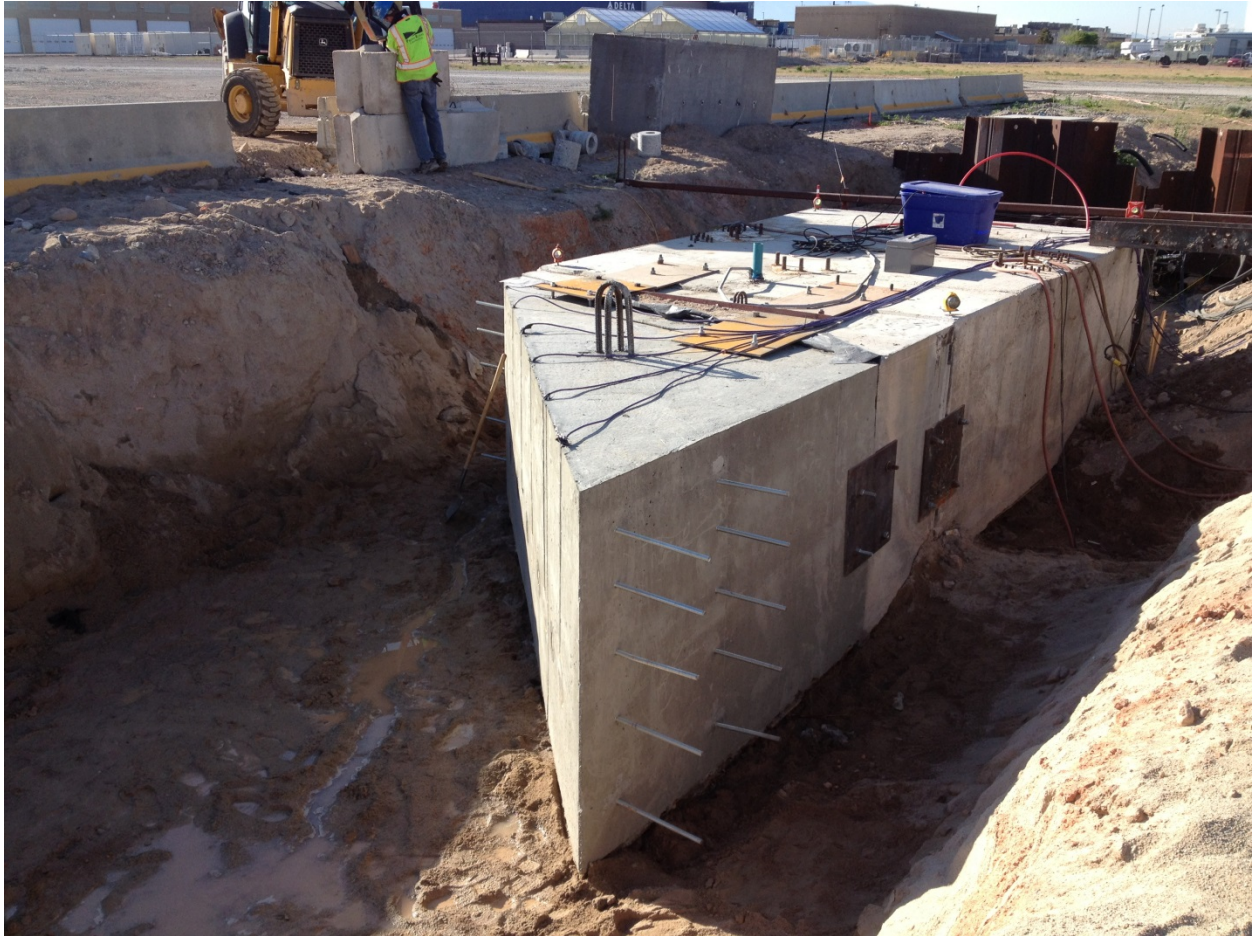
Figure 3.9. 45° skewed test abutment with threaded rod for securing wingwalls.
