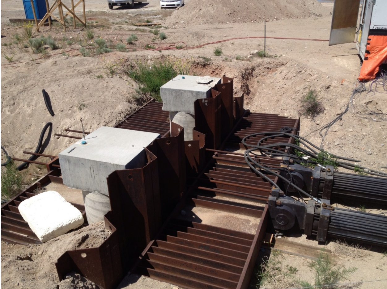
Figure 3.6. Reaction foundation for large-scale testing.
