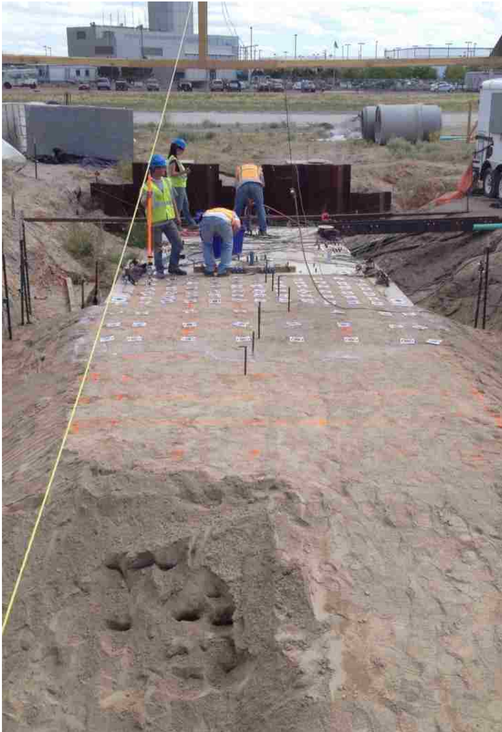
Figure 3.37. Backfill surface grid for non-skewed abutment.
