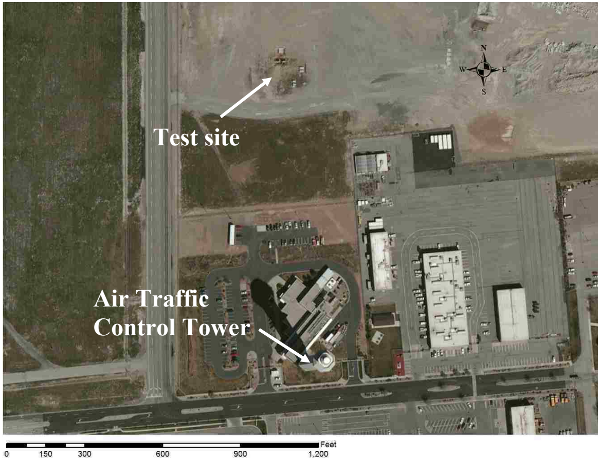
Figure 3.1. Large-scale field test site near Salt Lake City air traffic control tower.
