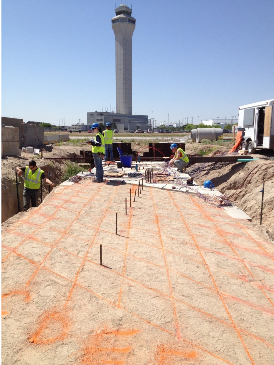
Figure 3.36. Orange spray-painted 2-ft grid on backfill surface for 45° skew.
