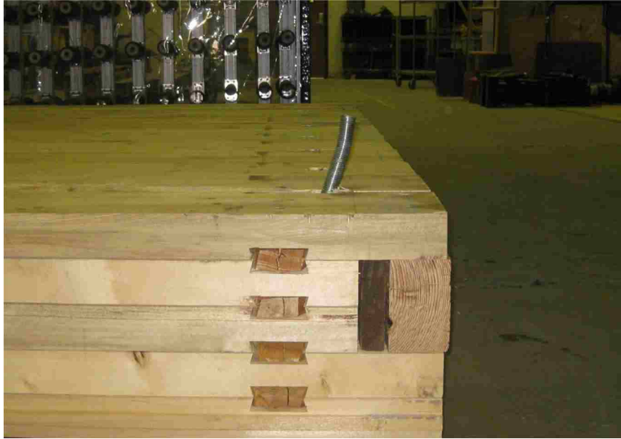
Figure B-6: Bottom Connection Bolt Bent from Testing (Wall 3)
