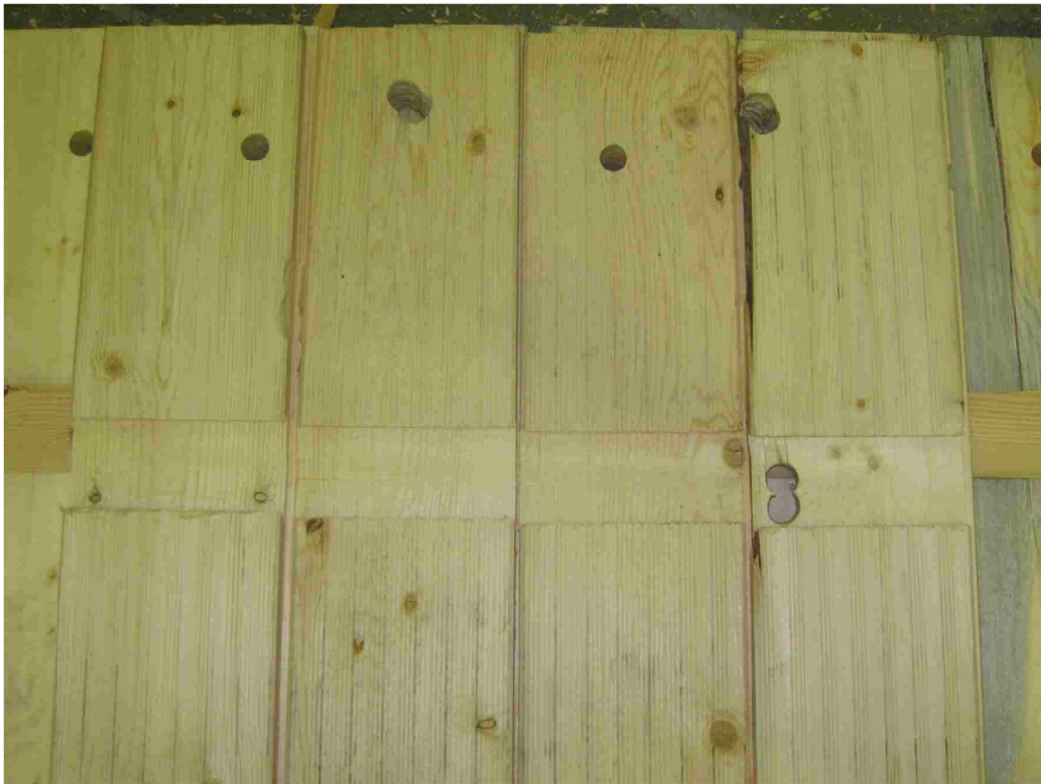
Figure B-4: Vertical Members with Dovetail Member Removed (Wall 2)
