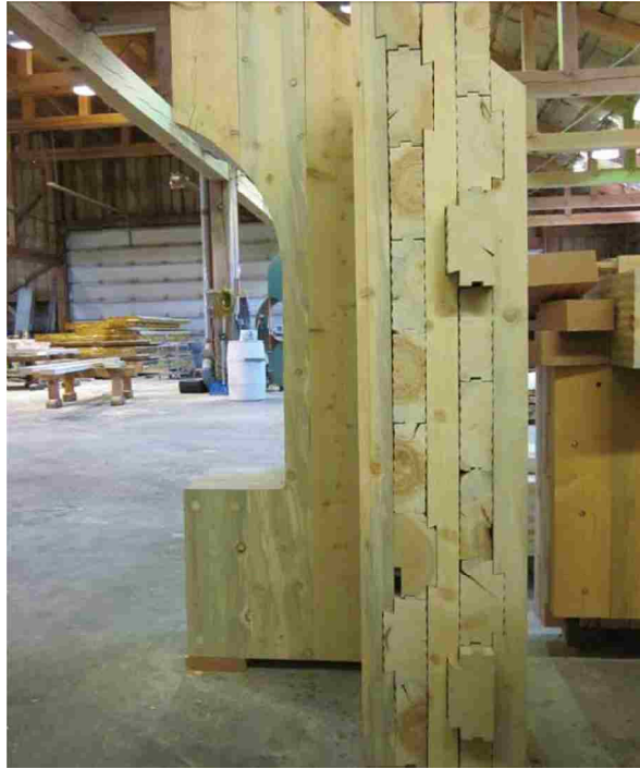
Figure 2-3: Cross Section of ICLT Panel (Apostol 2011)
