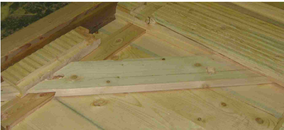
Figure 4-10: Diagonal Member with No Visible Deformations (Wall 3)
