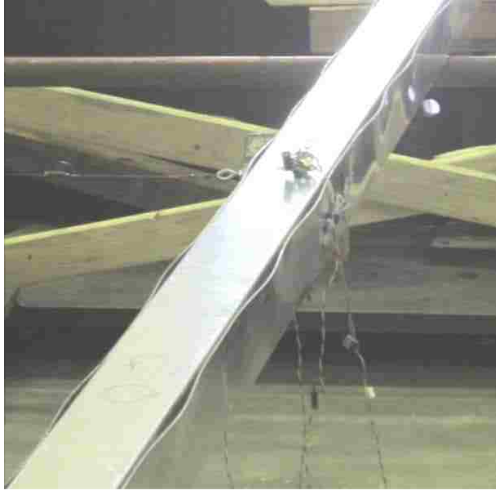
Figure 5-1: Photo of Local Buckling of “Adhesive-Only” Column During Test to Failure
