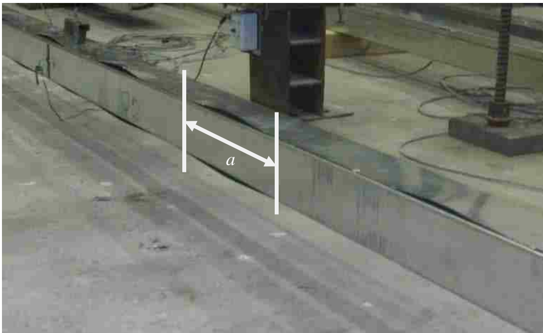
Figure 7-10: Close-up Photo of Local Buckling in “Adhesive-Only” Column During Test to 20 kips
