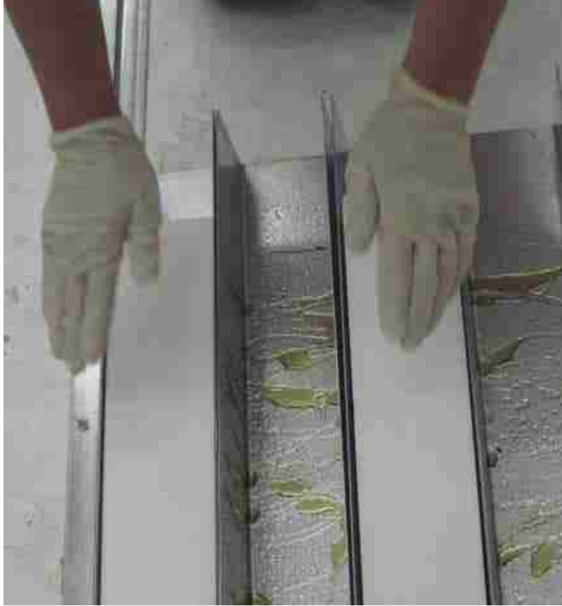
Figure 2-2: Photo Showing Fabrication of Columns: Insertion of EPS32 Foam into Steel Columns
