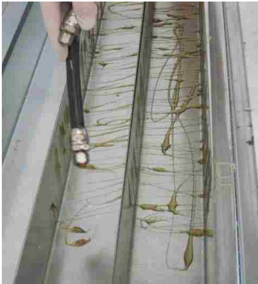
Figure 2-1: Photo Showing Fabrication of Columns: Application of Isogrip 4005D Adhesive
