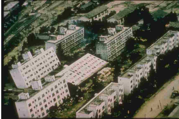
Figure 2-11: Bearing capacity failure after NOAA/NGDC - NOAA National Geophysical Data Center.
