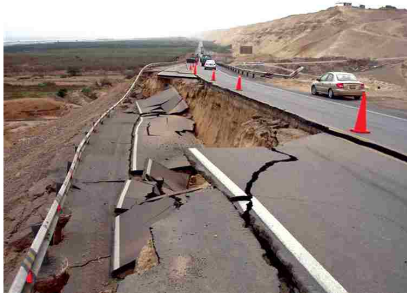
Figure 2-13: Retaining wall failure due to liquefaction after http://mceer.buffalo.edu/publications/bulletin/07/21-03/images/05embankmentlg.jpg .
