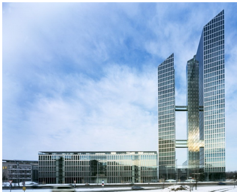
Figure 2-5: Highlight Towers (Architectism 2011)
