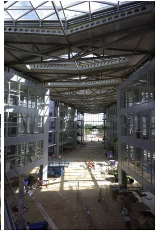
(b) Atrium Trusses
