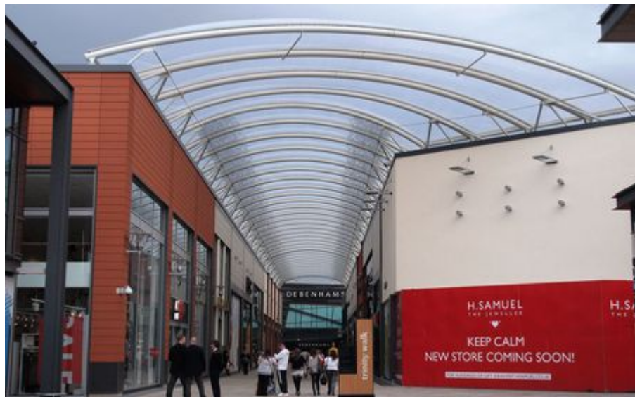
Figure 2-31: Trinity Walk Shopping Center (Architen 2011)
