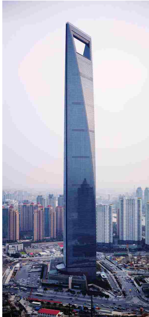
Figure 2-11: Shanghai World Financial Center (Architect 2009)
