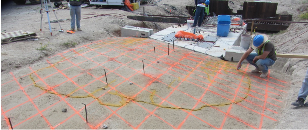
Figure 7-13: Completely developed failure wedge for the 30° test
