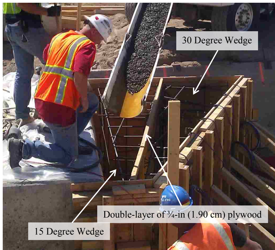
Figure 3-4: Simultaneous casting of 15° and 30° wedges
