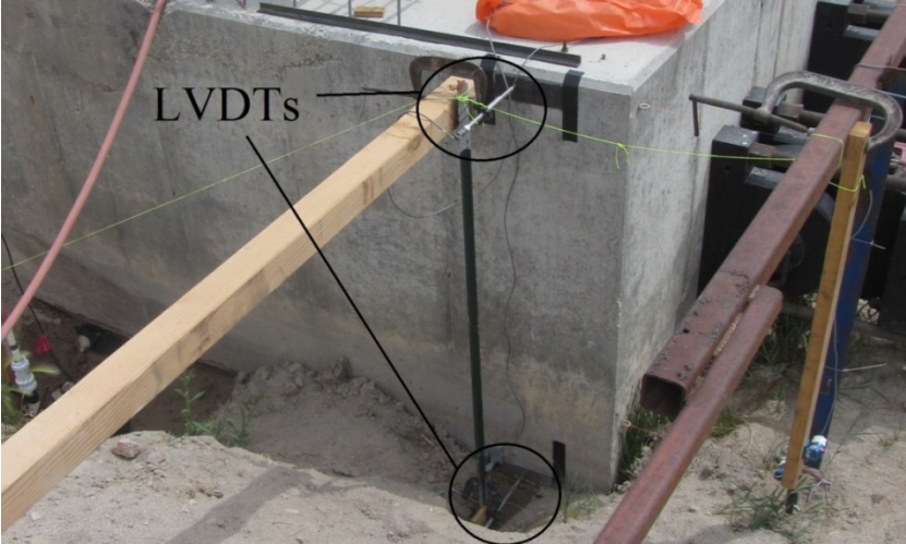
Figure 3-16: LVDTs for measuring transverse cap movement (south end)
