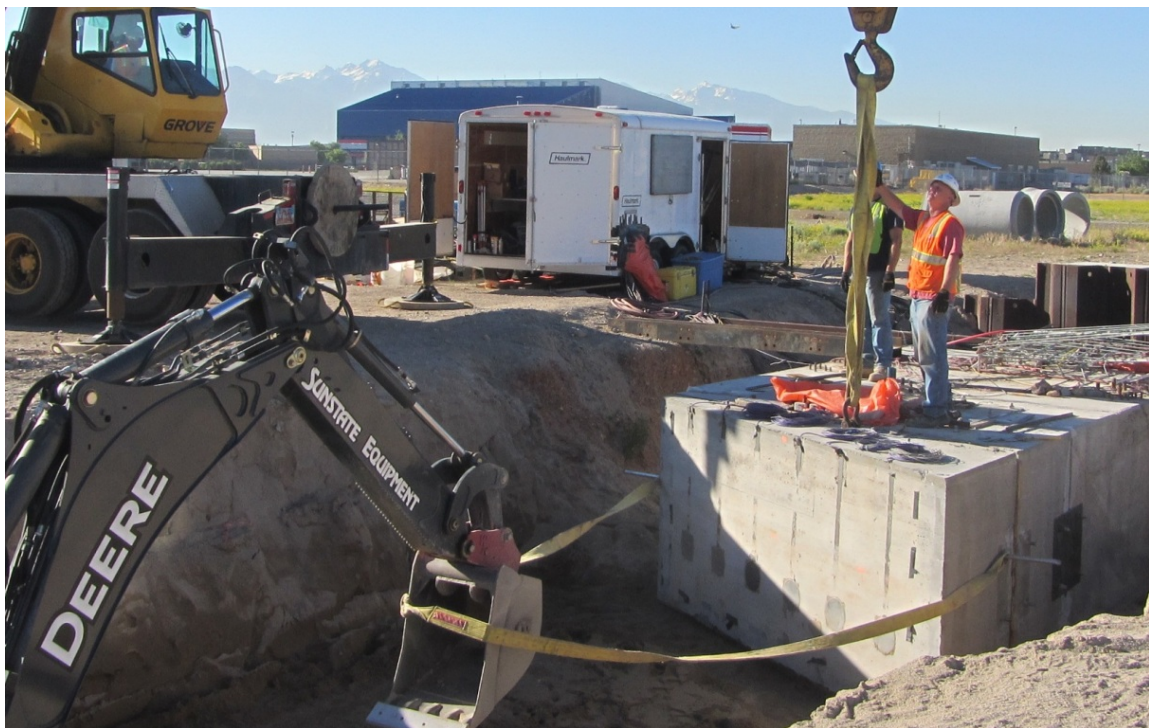
Figure 3-12: Removal of 30° wedge
