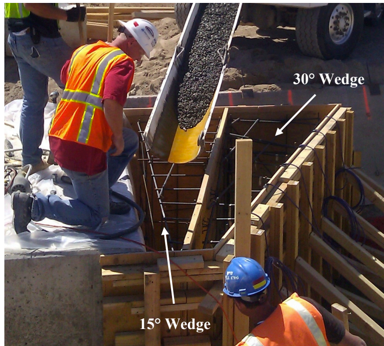
Figure 3-4: Casting of 15° and 30° wedges
