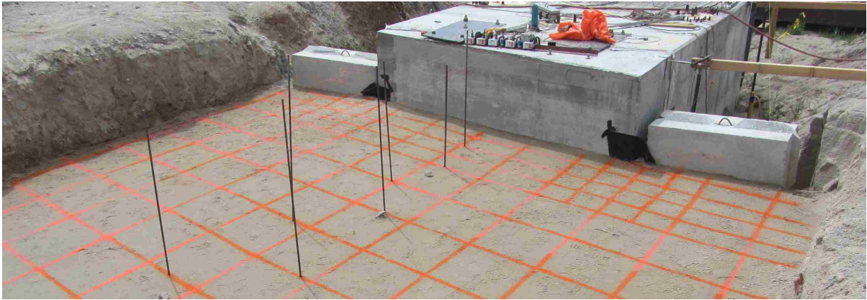
Figure 3-14: String potentiometer setup for backfill movement and strain measurements
