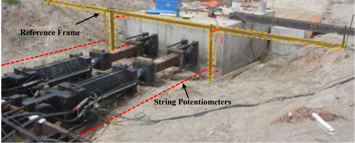
Figure 3-13: String potentiometer locations on south end of pile cap
