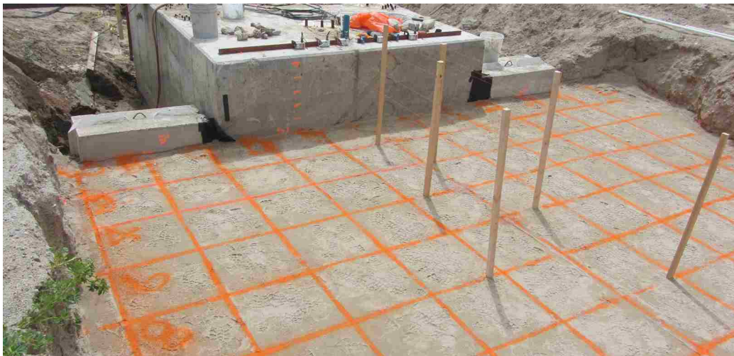
Figure 3-34: Backfill surface fully prepped for testing
