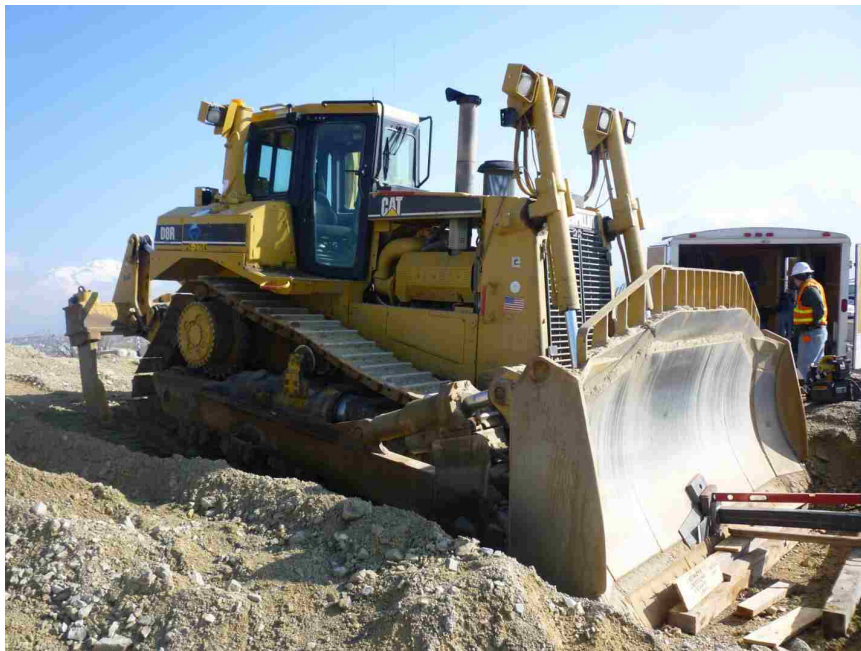
Figure 5.5: Equipment used to react load at TP4 from 0.75 to 3.5 in. displacement, and all load at TP5 (Pioneer Crossing Site).
