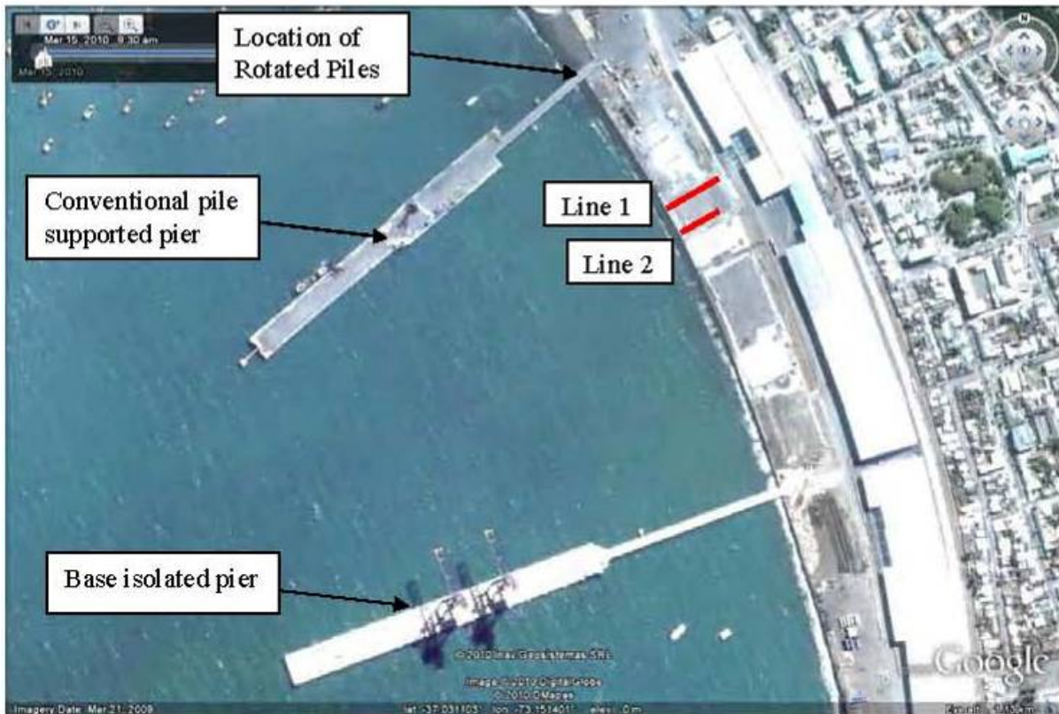
Figure 5-2: Location of North and South Piers. Photo from (GEER 2010)
