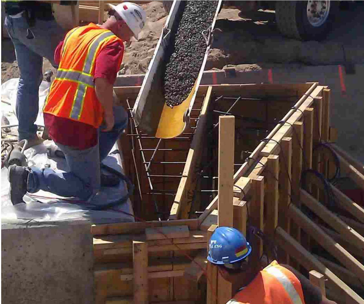
Figure 3.6: Simultaneous Casing of the 15° and 30° Wedges
