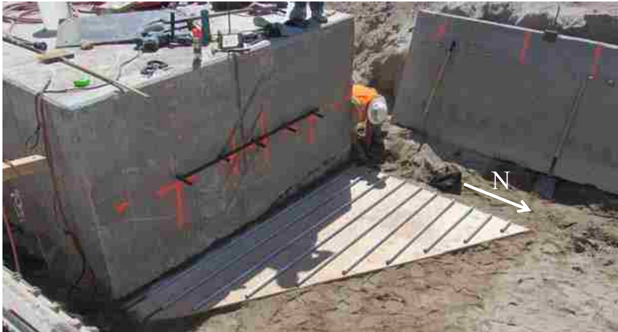
Figure 3.11: Steel Roller Bearing Platform for Concrete Wedges
