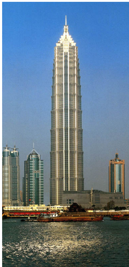
Figure 1-1: Jin Mao Tower – Shanghai, China © SOM
