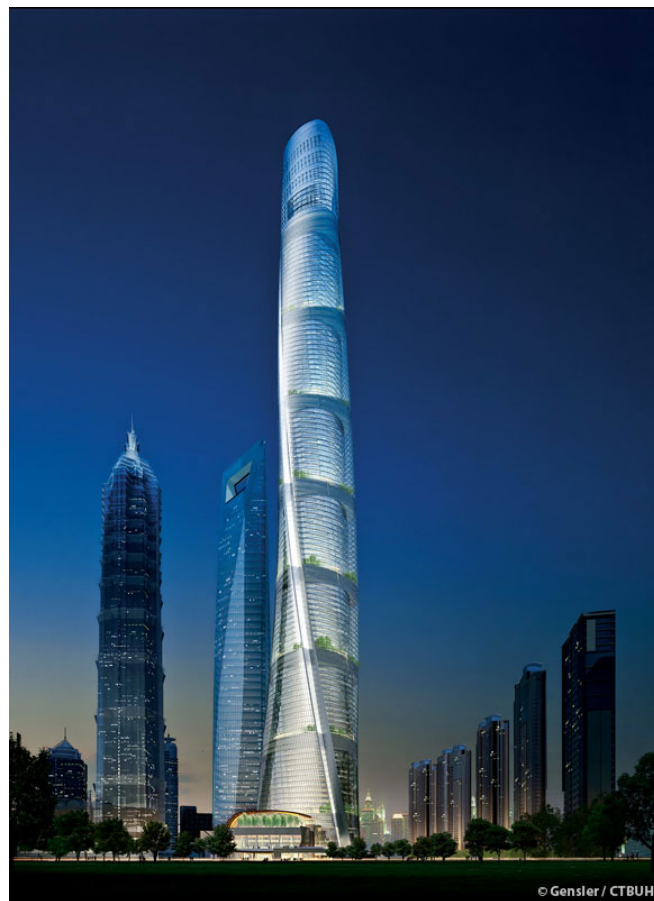
Figure 1-7: Shanghai Tower © Gensler
