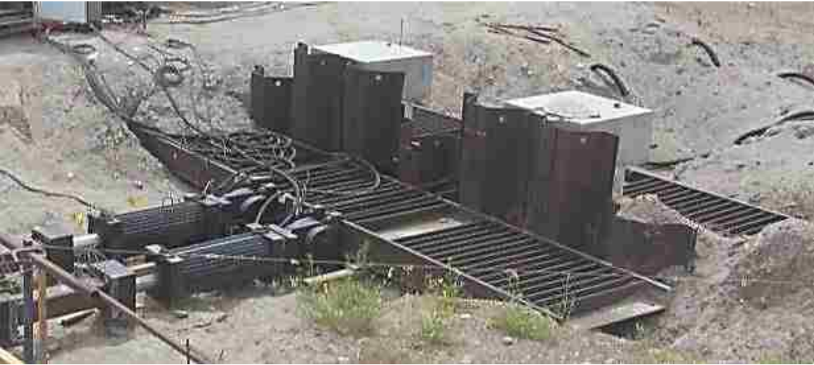
Figure 3.8: North side of reaction foundation
