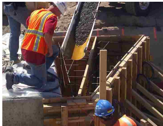
Figure 3.10: Construction of 15° and 30° wedges (Marsh 2013)
