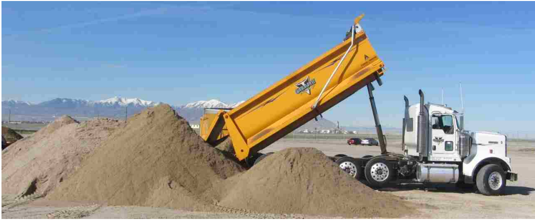
Figure 3.13: Delivered backfill sand (SP)
