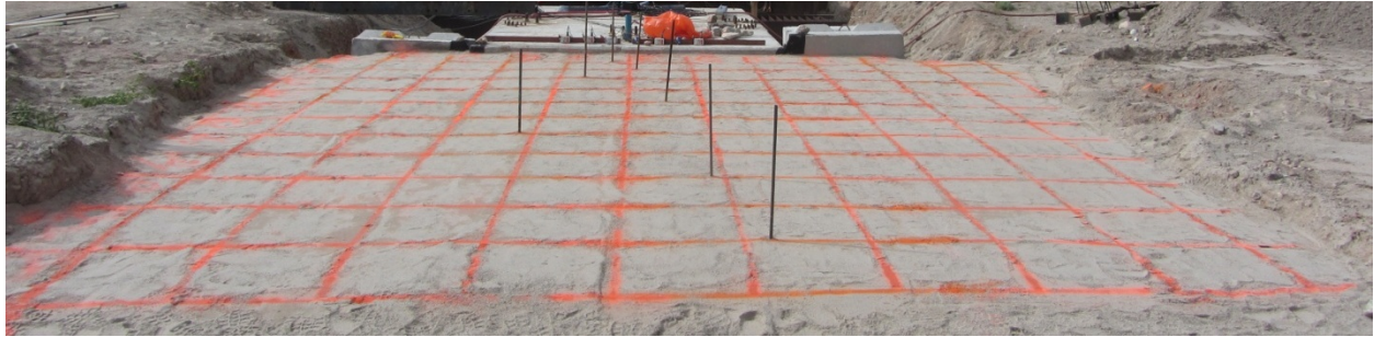
Figure 3.30: General backfill surface grid
