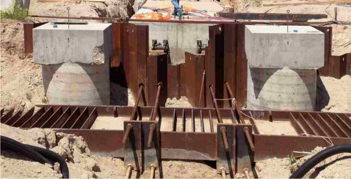
Figure 3.7: South side of reaction foundation
