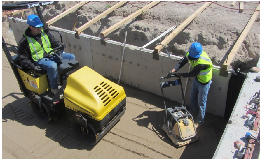
Figure 3.28: Compaction instruments with vibrator roller compactor on left and plate compactor on right
