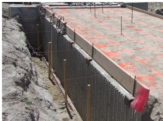
Figure 3.25: MSE wall instrumentation setup for 0° test
