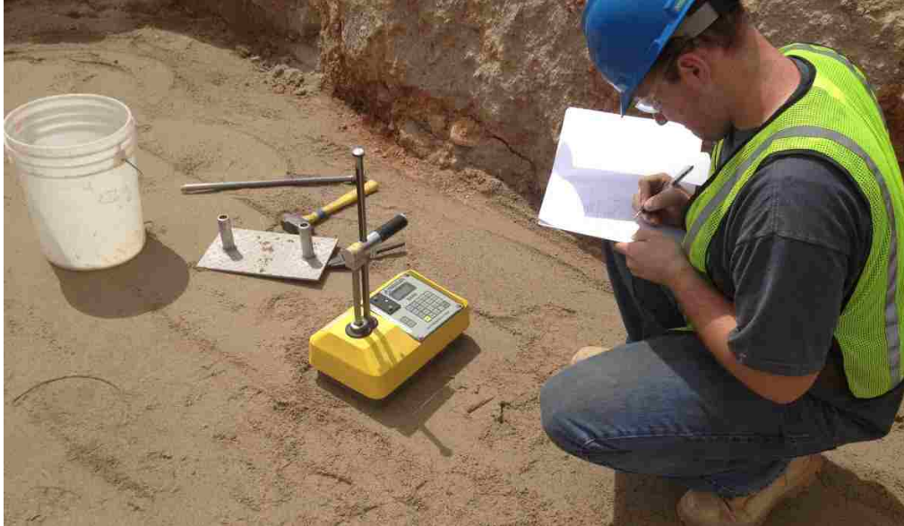
Figure 3.29: Testing soil with nuclear gage
