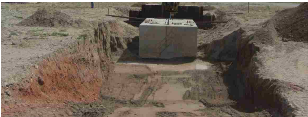
Figure 3.12: Test site backfill zone
