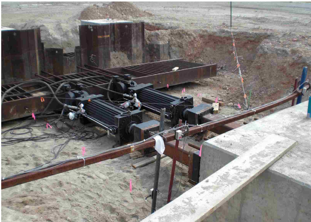
Figure 4-2: Picture of string pots from reference frame to load frame.
