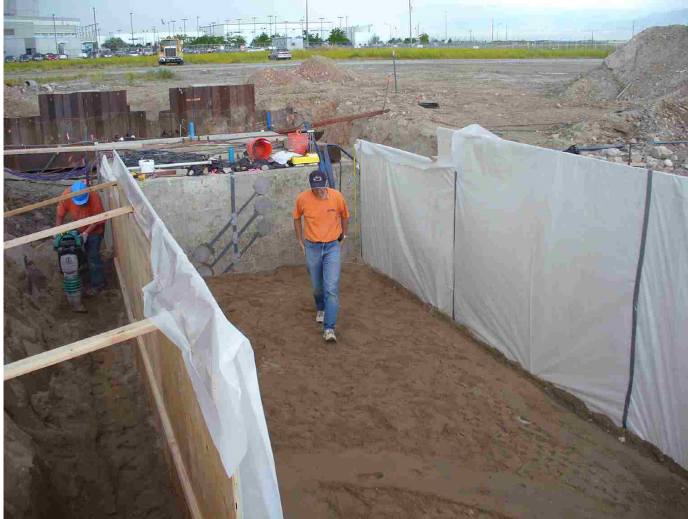
Figure 4-8: Picture of side isolation panels being backfilled.
