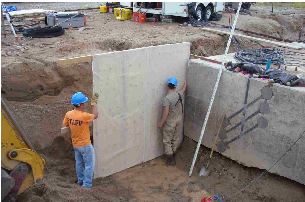
Figure 4-7: Installation of side isolation panels.
