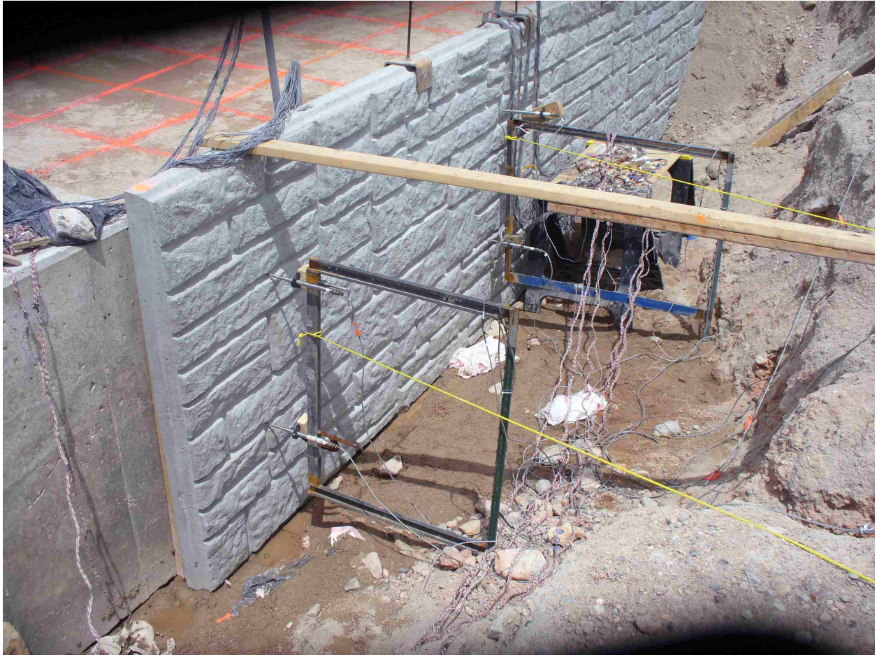
Figure 4-18: LVDT's to measure wall deflection.
