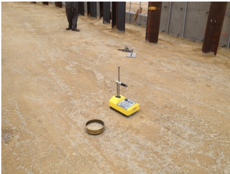
Figure 3-7: Nuclear Density Gauge Testing
