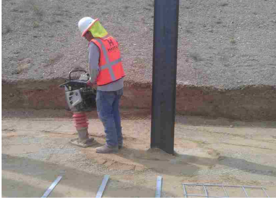
Figure 3-6: Jumping Jack Type Compaction Around Test Piles Investigated in This Study
