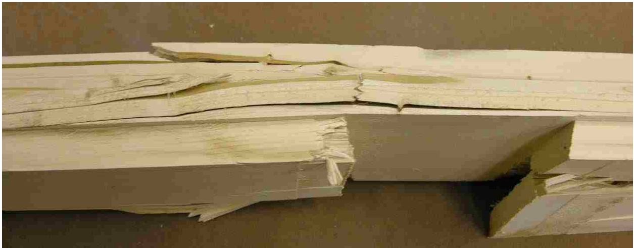
Figure C-4: Typical Buckling Failure of Vertical Members in Compression Wall
