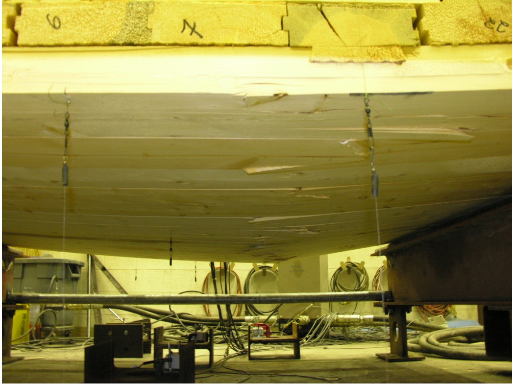
Figure B-2: Failure of Underside of Flexural Wall
