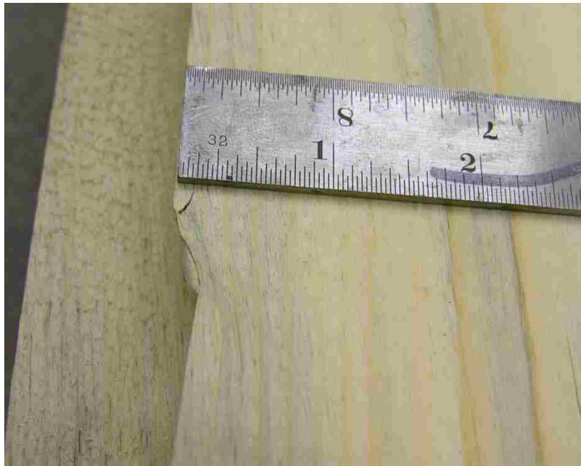
Figure A-6:Measured Crushing of Dovetail Section in Racking Wall
