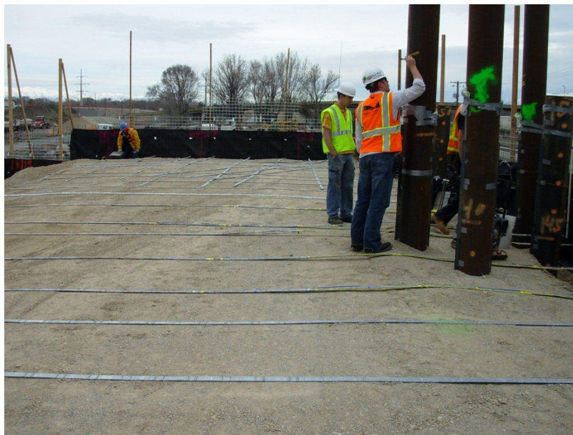
Figure 3.1: Test piles with bottom instrumented layer of steel strip reinforcement
