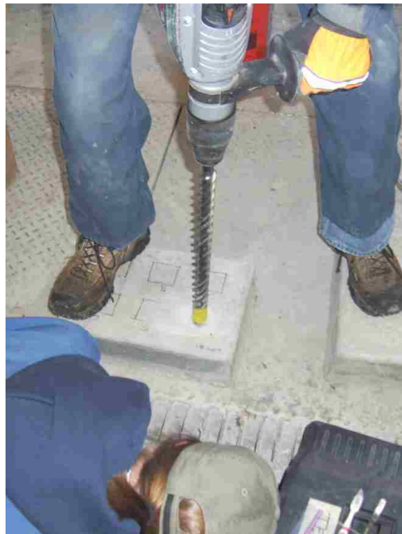
Figure 3-10: Drilling a slab.
