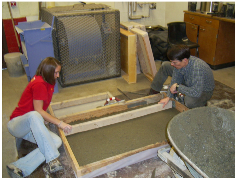
Figure 3-4: Screeding a lift.
