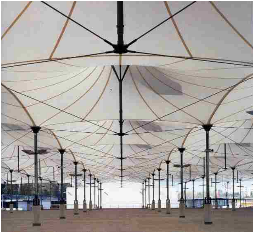
Figure 34: Cable-Strut System Supporting the Membrane between Columns
