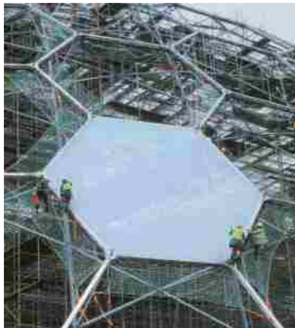
Figure 24: Installation of ETFE Cushion
