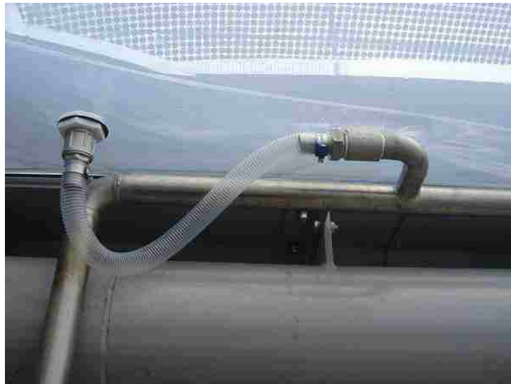
Figure 3: Air Hose Connection to an ETFE Cushion.
