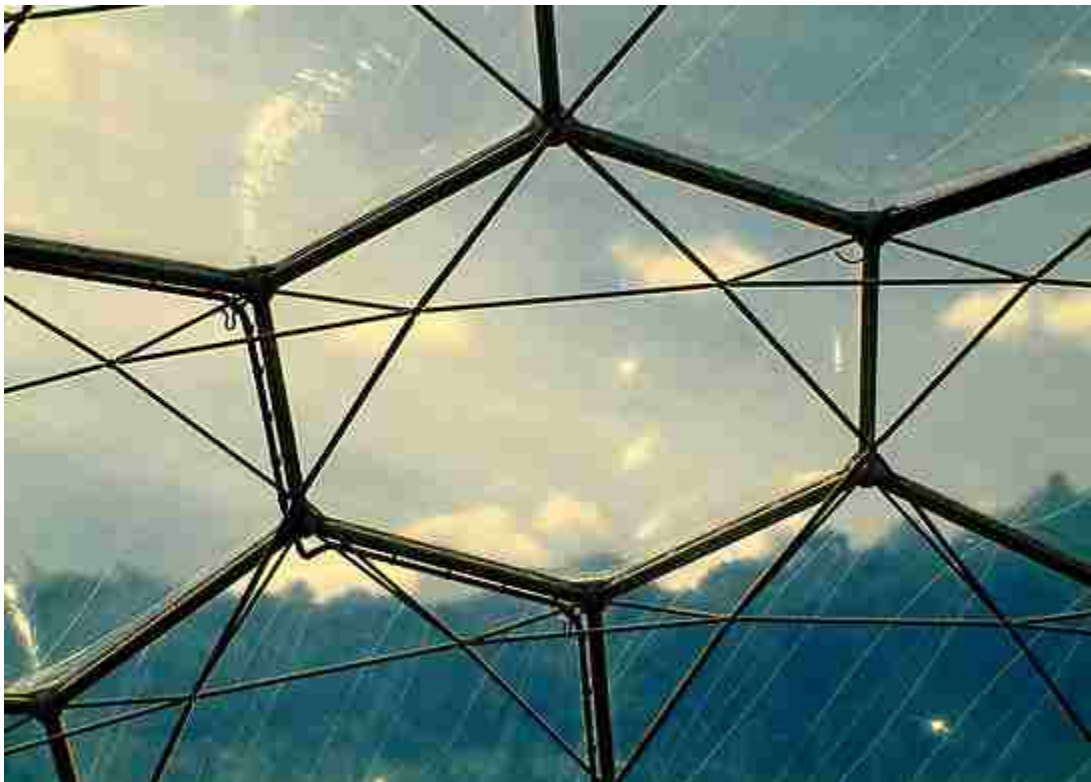
Figure 23: Close Up of Double Layered Space Frame
