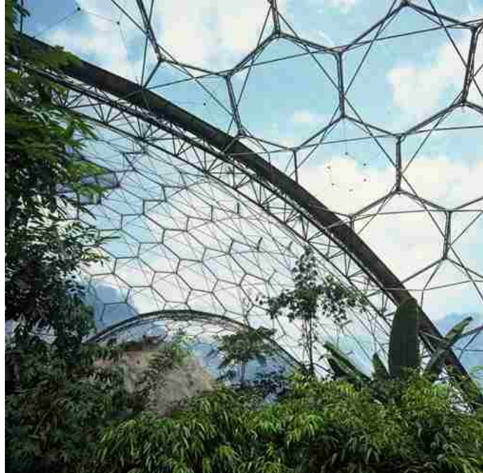
Figure 26: Arched Trusses and Cable Nets.
