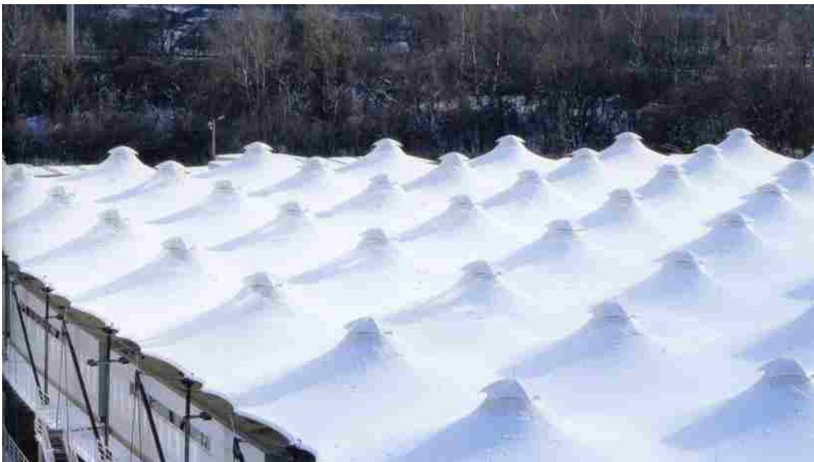
Figure 33: Exterior of Truck Depot
