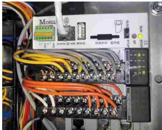
Figure 5: Cushion Pressure Control System
