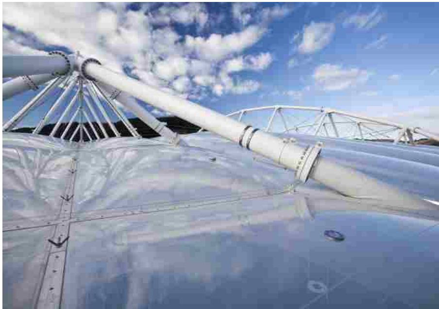
Figure 44: Close Up of Trusses and Connections
