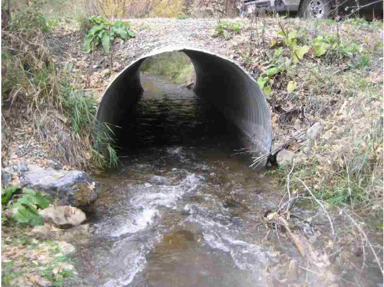
Figure 3-10: South Fork Culvert from Upstream Reach Looking Downstream.
