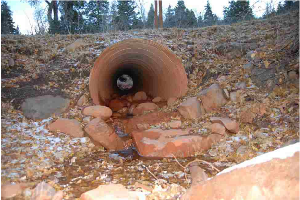
Figure 3-4: Red Creek Culvert Downstream Invert Looking Upstream.
