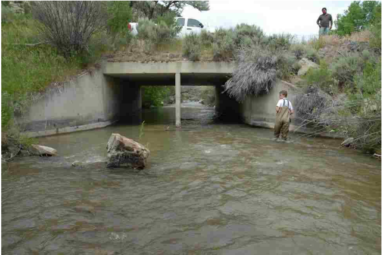
Figure 3-6: Salina Creek Culvert from Upstream Reach Looking Downstream.
