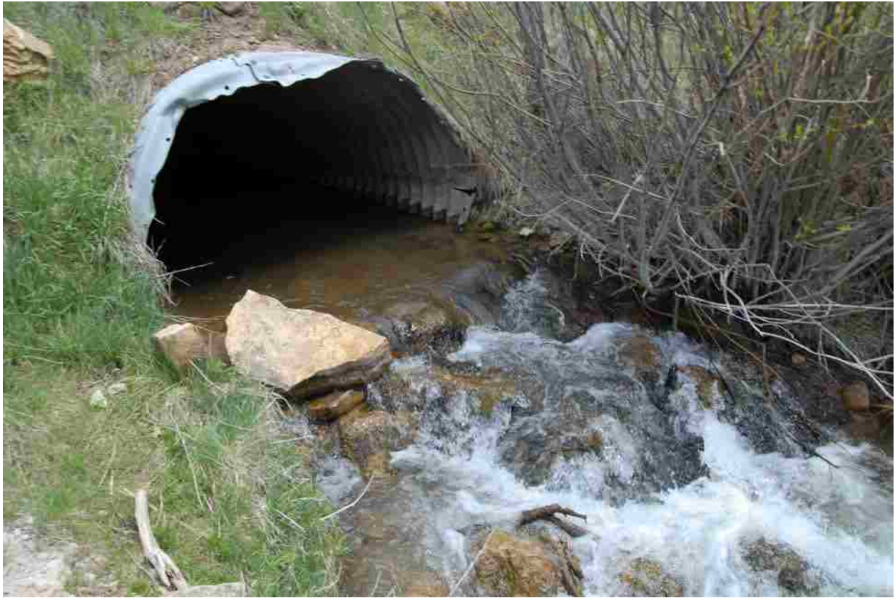
Figure 3-2: Hall's Fork Culvert Downstream Invert (Photo taken by Ryan Woods).
