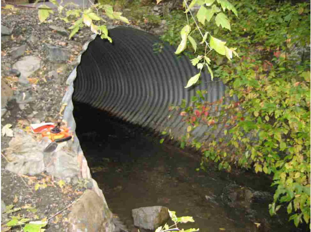
Figure 3-12: Summit Creek Culvert Downstream Invert.
