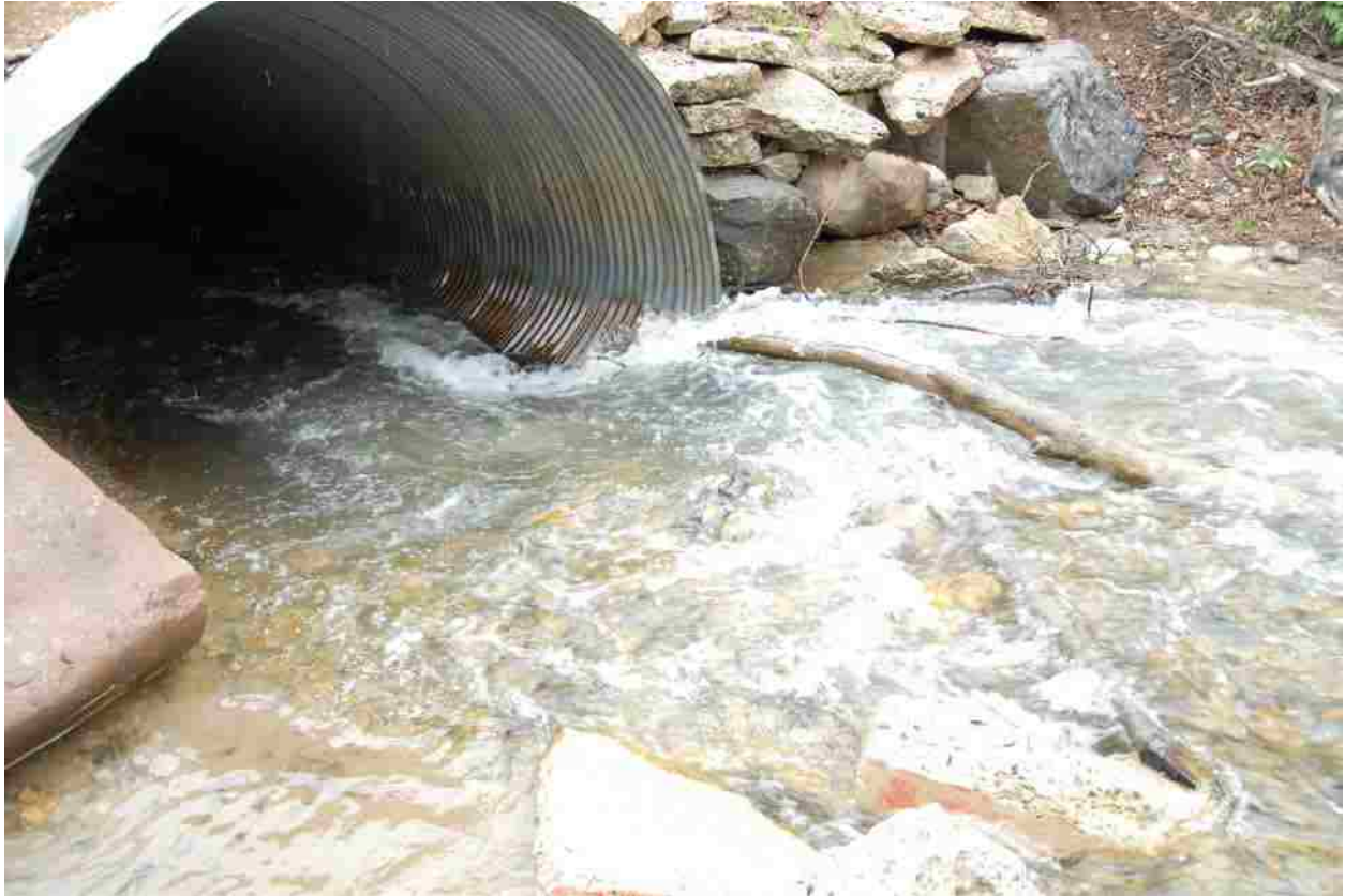
Figure 3-8: Salt Creek Culvert Upstream Invert.
