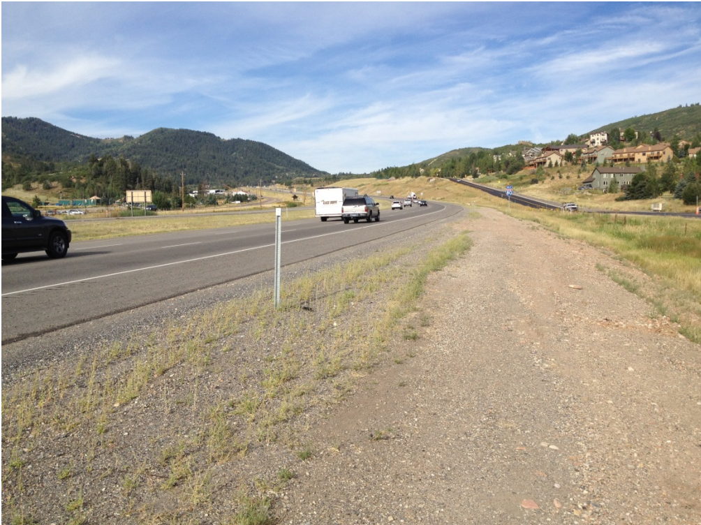
Figure 6-8: Typical shoulder on Interstate 80.
