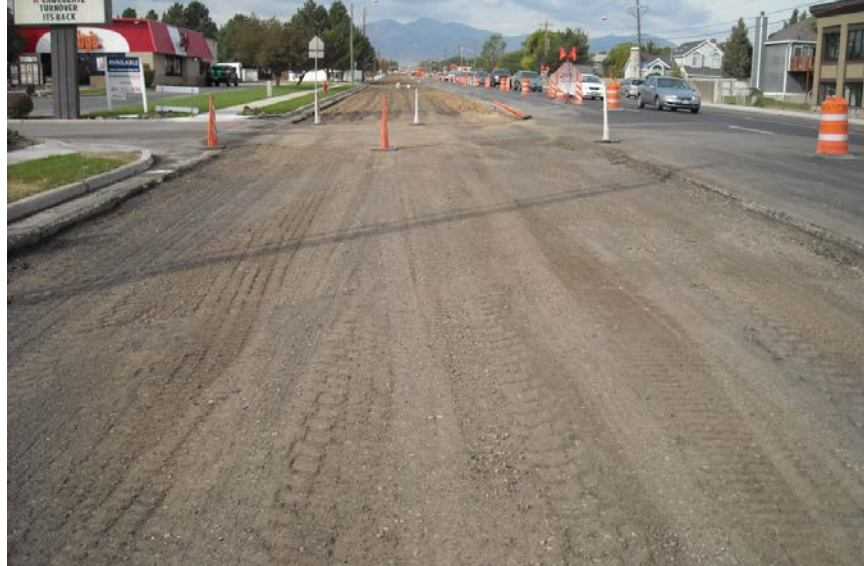
Figure 3-1: Base material prepared for emulsion treatment.
