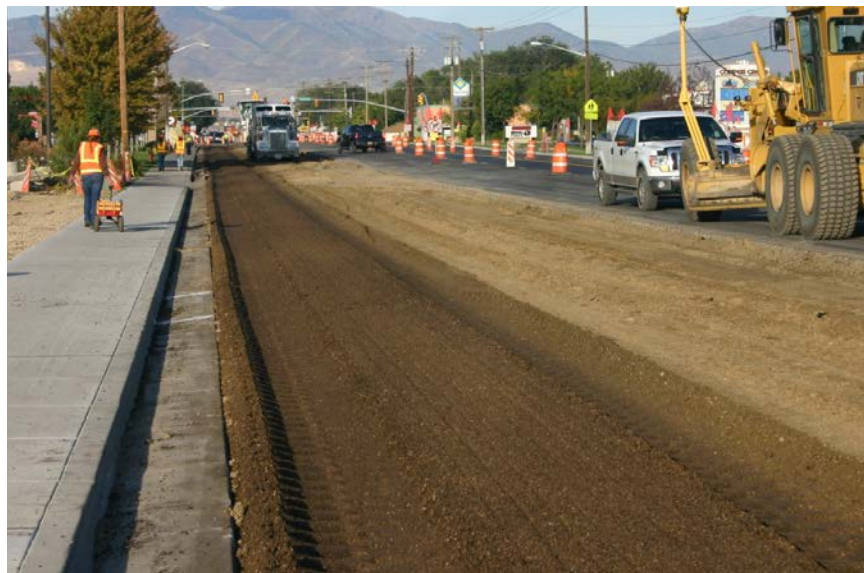
Figure 3-2: Emulsion treatment of prepared base material.
