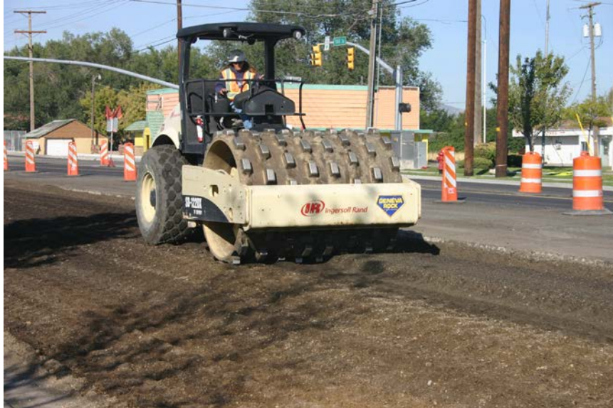
Figure 2-3: Emulsion-treated base compaction.
