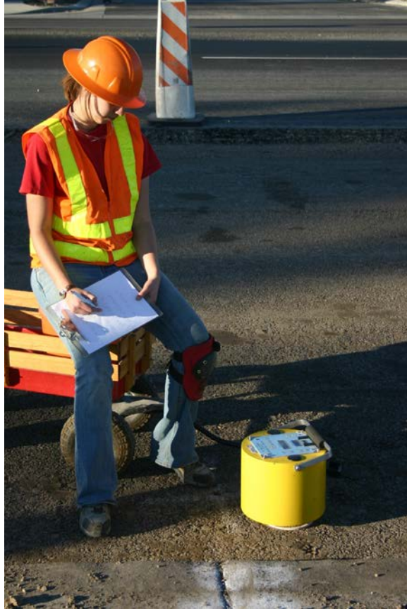
Figure 3-7: Soil stiffness gauge.
