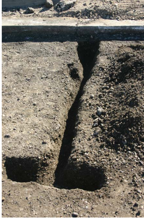
Figure 3-15: Sensor site just before installation of sensors.
